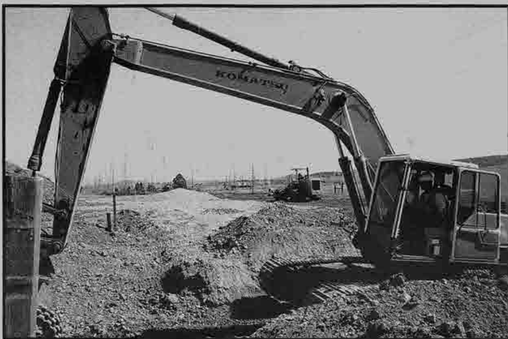
Above: Excavator Operator Steve Julian, using a compactor attachment, works on backfilling a utility trench at Broadstone.
