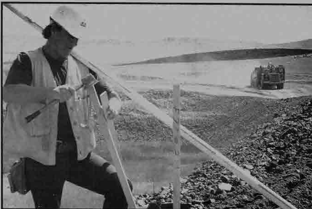
Gradesetter Sam Vassy works near the fill area at Broadstone, where crews moved a total of 850,000 yards, much of it hard shale and granite.
