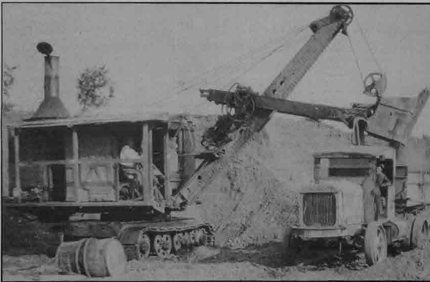
Top: Gene operated this Brownhoist No. 2 crane in 1923 at the E.B. & A. L. Stone gravel plant in Coyote near San Jose. The old clamshell, powered by a 60 horsepower gasoline motor, had horizontal operating levers.
