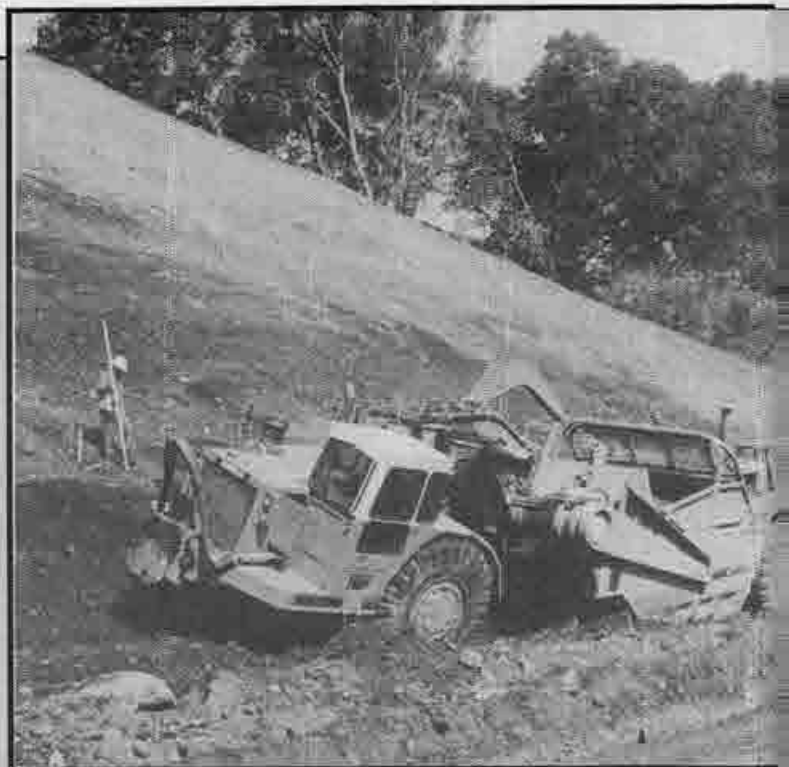
Top center: These 657 scrapers are moving most of the job's 1.3 million Top right: C. A. Rasmussen's crew.
