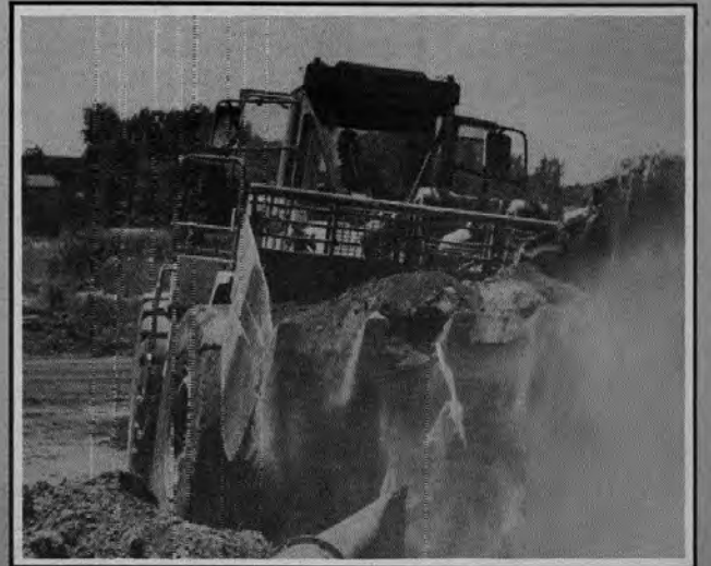
Master mechanic Mike Lange (far left) checks out the Holland Loader for Ball, Ball & Brosamer during lunch break. Pictured immediate left on backhoe is Joe Gruhl. Andy Cook (above) clears away overburden with Cat 988 loader. Workers make a major concrete pour (right) on Gibbons & Reed contract at 5th South & I-215.
