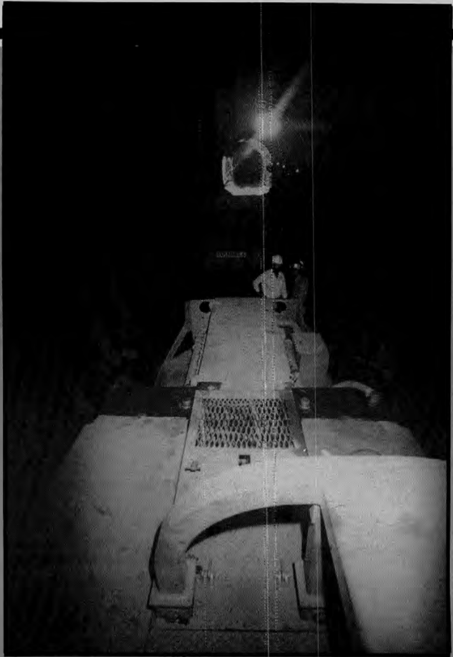
View of main tunnel section with east portal in distance.
