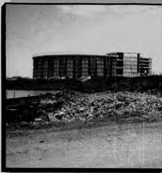
Waikoloa Hyatt Pictured on this page is the Waikoloa Hyatt project, under construction in Kona by general contractor Hawn Dredging. Sub-contractor on the job is Goodfellow Bros.
