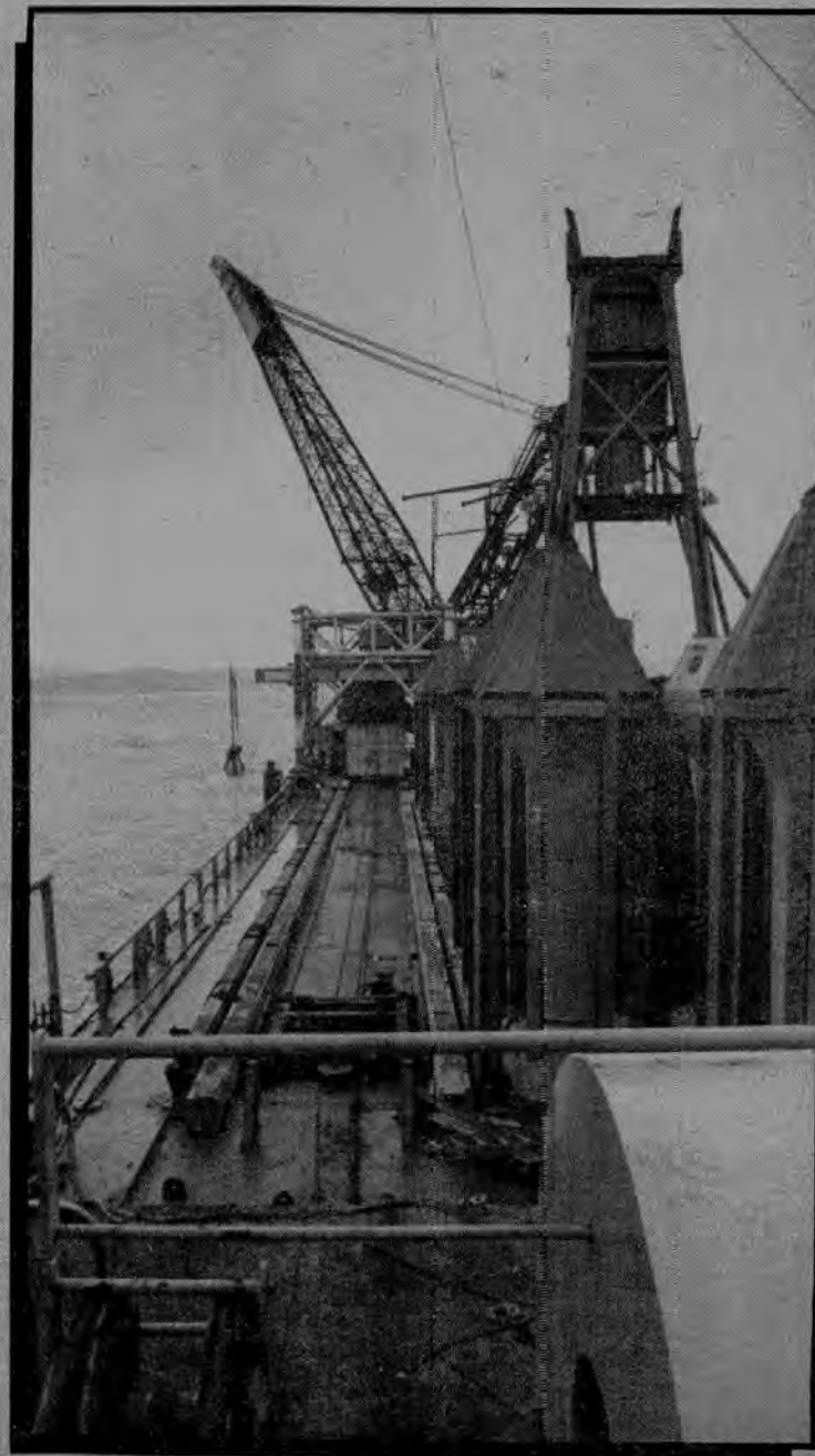
Getting to work on the ocean outfall job was not the normal commute for Local 3 members. The 'Betty L' (top left) is equipped with a helicopter landing pad to carry workers on and off board. On deck of the 'Betty L' is the workhorse of the barge, a 500-ton Clyde Crane (above).
