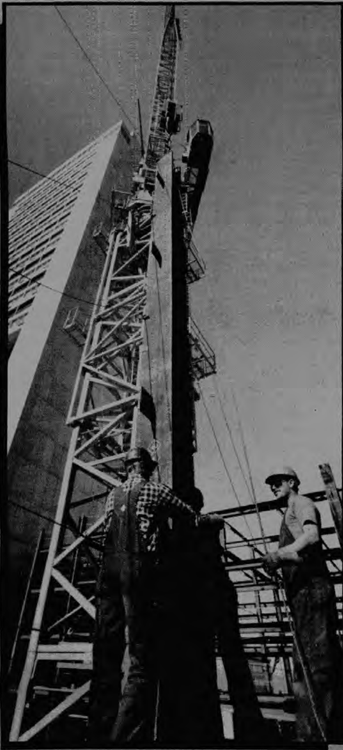
Local 3 tower crane operator Sam Timas (top right photo) demonstrates how the weight of each load is given on a digital readout. Ironworkers (above) ready a column for a lift on the 28-story Hilton Tower project in San Francisco. Below, the Liebherr crane's boom seems to converge on the existing Hilton tower in the wide angle photo.
