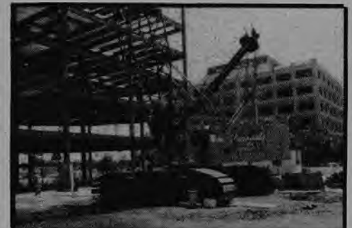
Prototype crawler crane in San Jose — pg. 9
