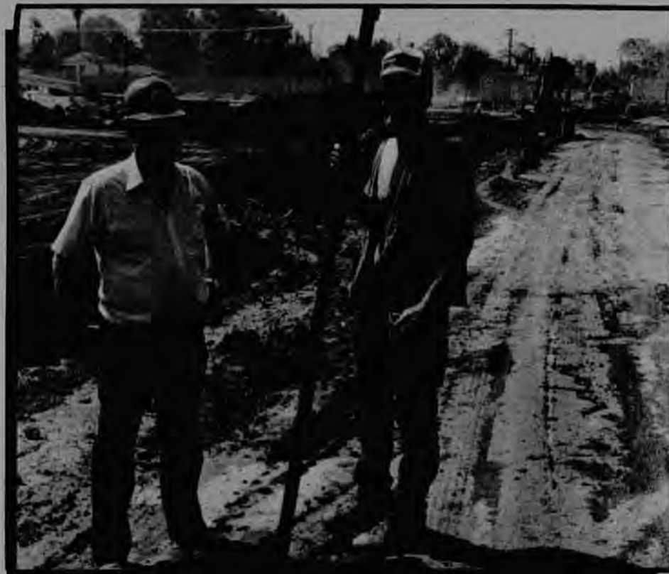
San Jose Business Agent Max Spurgeon is pictured above with gradechecker Joe Koehler on the San Jose convention center project.
