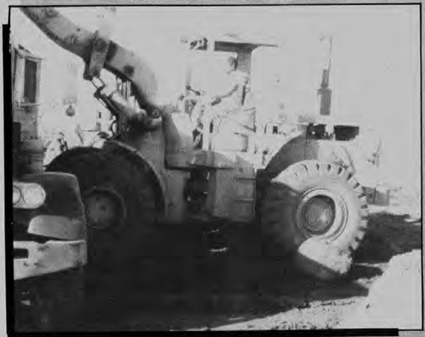
In the bottom photo, John Kuamoo runs a loader for Delta Construction on the Kaanapali Hillside project in Maui. Working on the same project (second photo from bottom), is Daniel Delima on a rubber tired blade.
