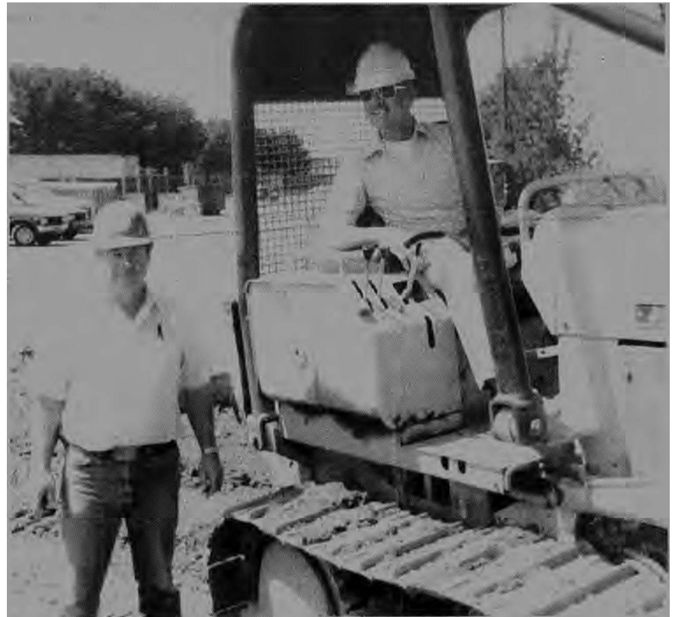
Laying pads for Optical Coating of Santa Rosa are Local 3 members Paul Heater (Grievance Committeeman) and Stu Orchard.
