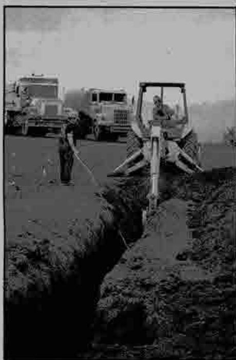
At the Kunia training center are Gilbert Kahaleauiki on the backhoe and William Nelson checking grade.
