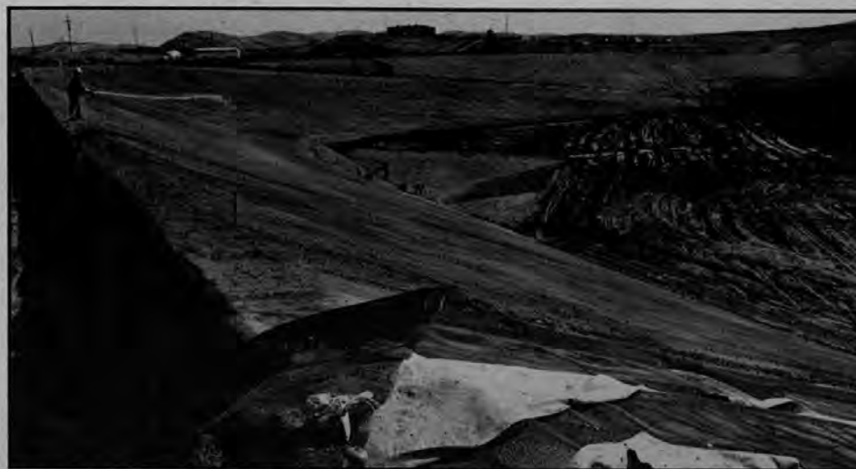
An impervious lining of clay, gravel and geosynthetic plastic will form the base of the new holding pond.
