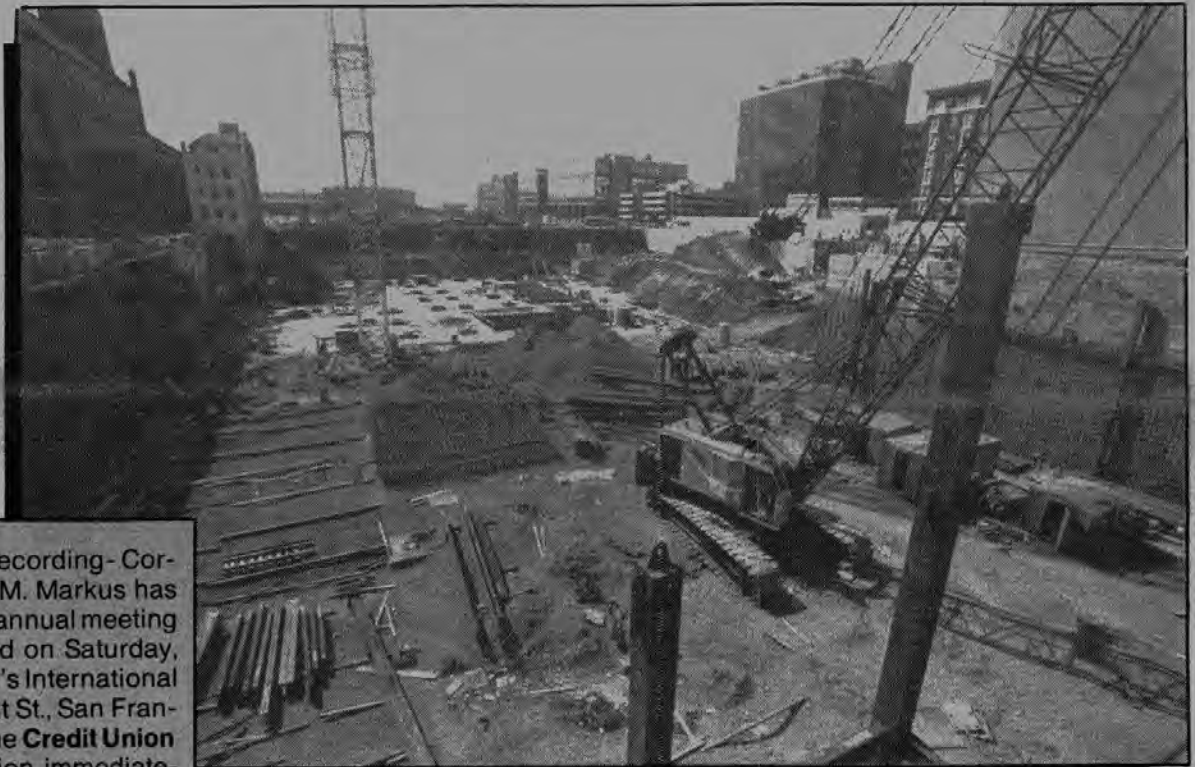
Workers begin steel erection on Yerba Buena's Marriott Hotel.
