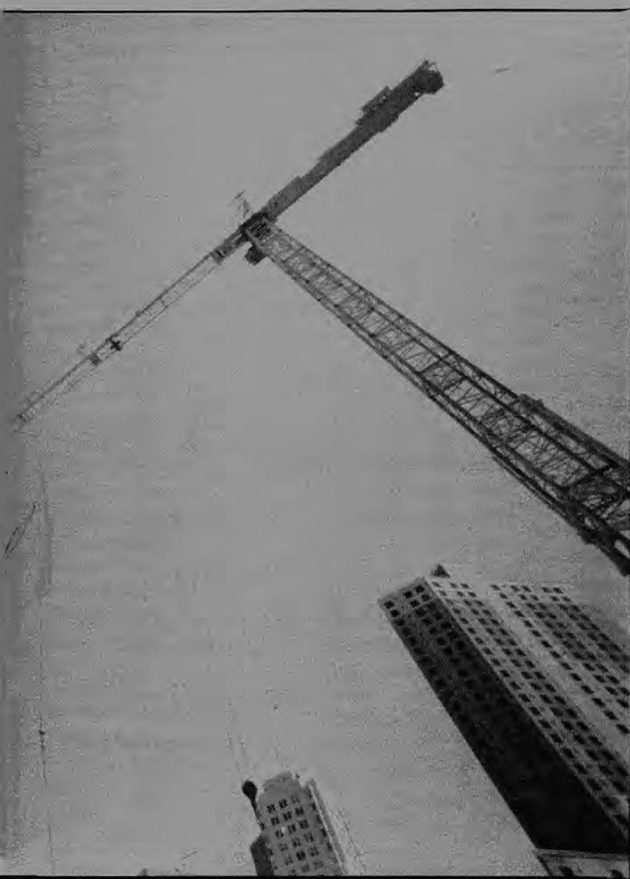
Operator Cathy Hilton sits high above the Marriott Hotel project.
