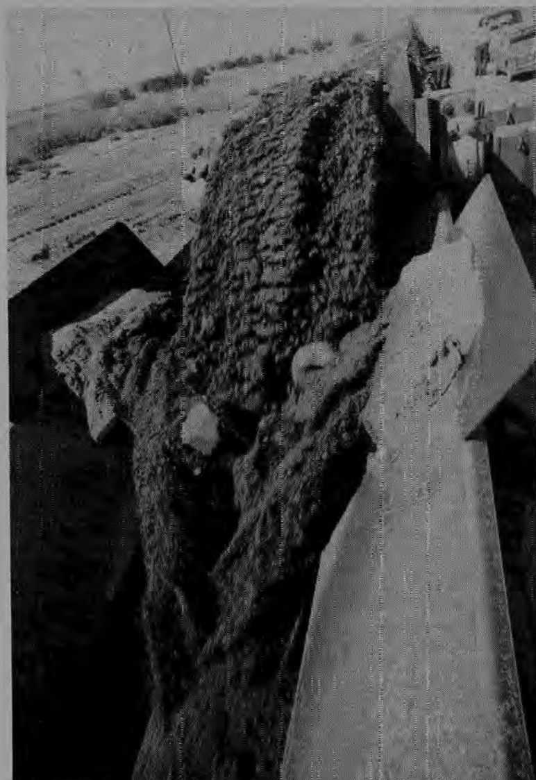
Dirt to be used for fill catapaults along a record-length 13-mile conveyor belt on S.J. Groves' $46 million I-80 job just west of Salt Lake City.
