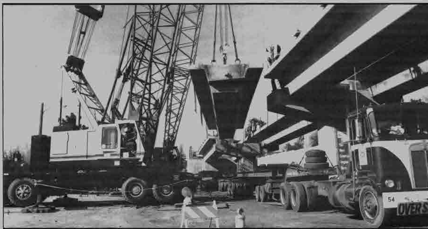
A section of aerial trackway is hoisted into place along the section that leads from the existing Concord station to the new North Concord-Martinez station.
