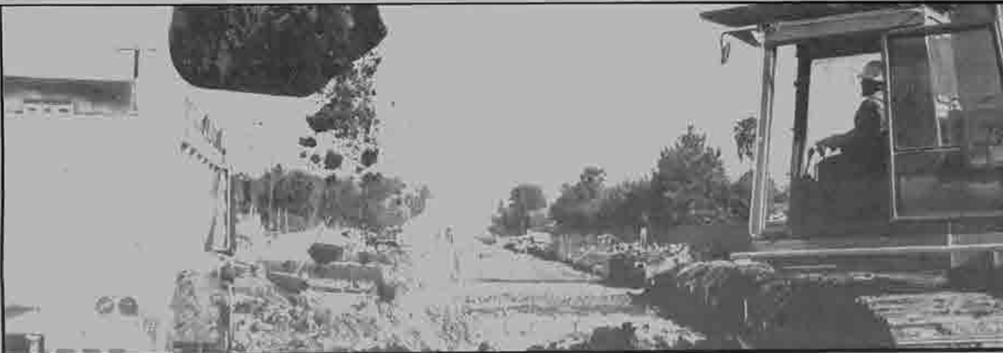
Left: Excavator operator Delmar Campbell digs hole for column foundations.
