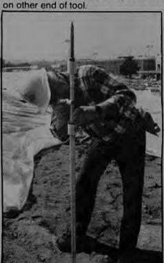
Tool can then be used to shoot grade with hand level.
