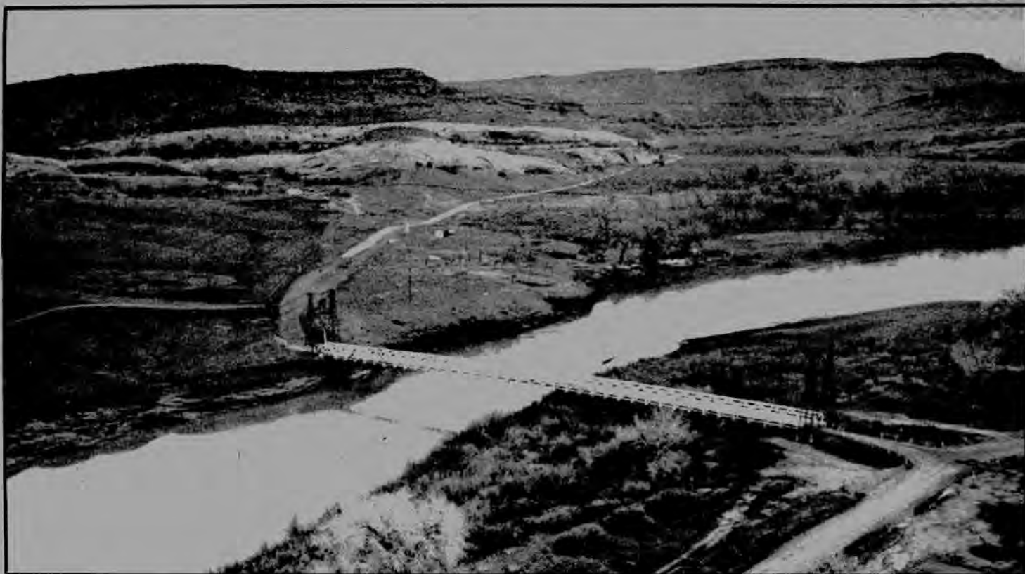
Pictured above is the old Dewey Bridge on Route 128, which is in the process of being replaced.
