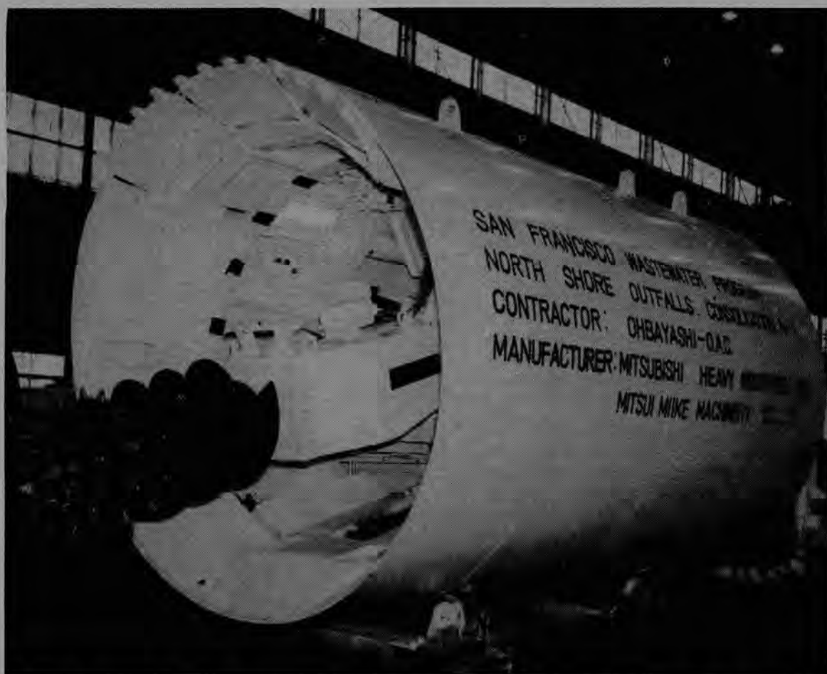
Pictured above is one of the two massive tunnel boring machines to be used in the $22 million tunnel job—part of the $1.5 billion San Francisco waste water treatment project. The contract was awarded to Ohbayashi-O.A.C.,
