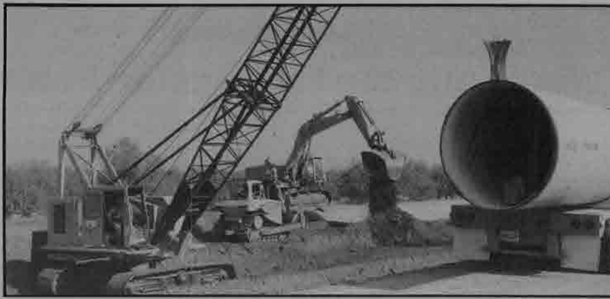
Left: The steel pipe was brought by truck and off loaded with cranes.
