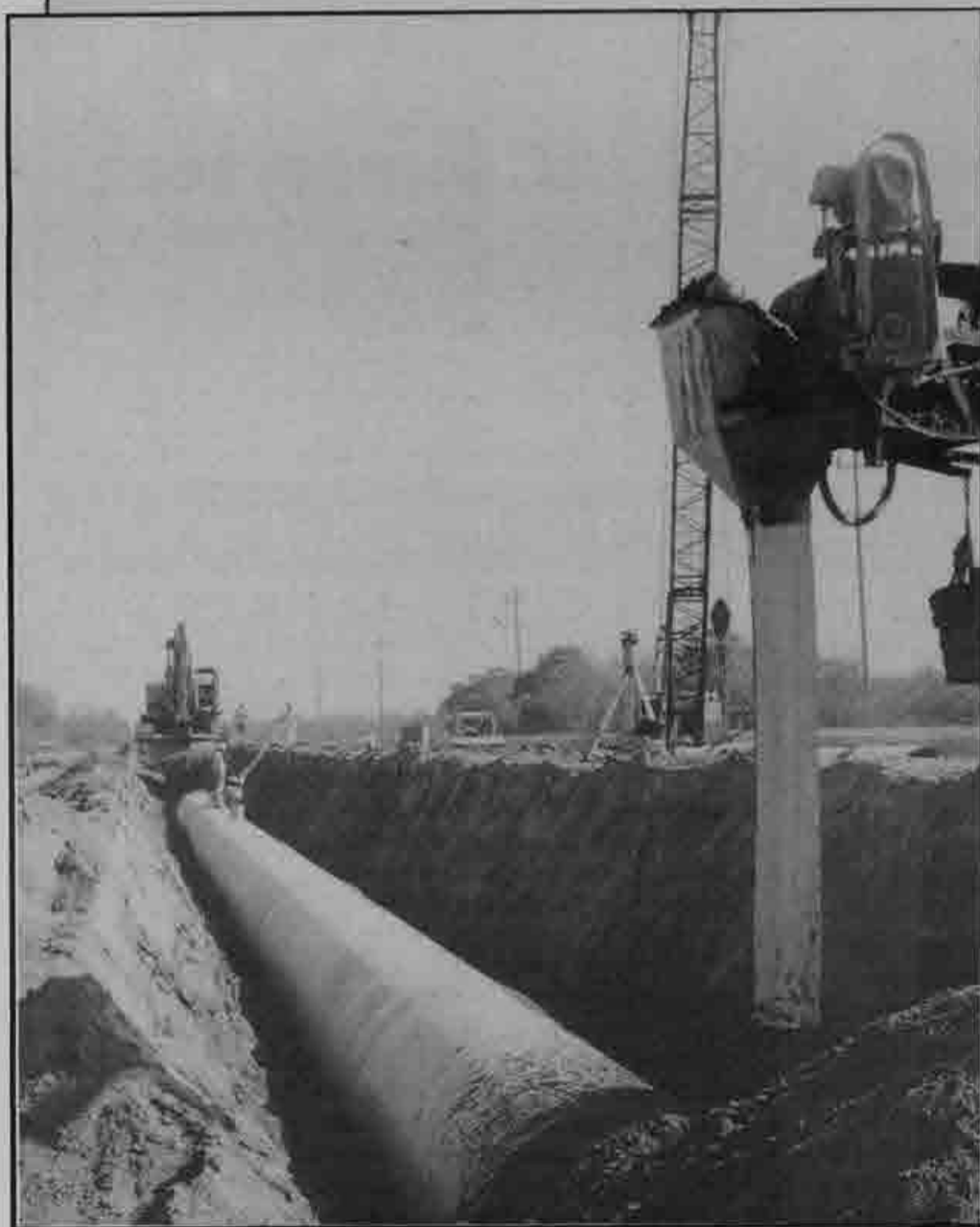
Top: Mountain Cascade's soil processor at work on Modesto Irrigation District's 16-mile water pipeline project.
