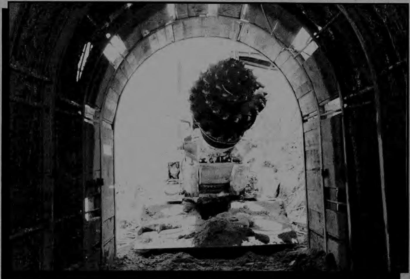
are designed to rotate as they cut to produce a longer lasting, even wear on the carbide tips.
