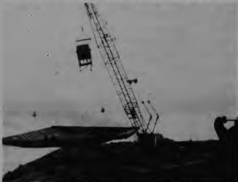
A 3900 Manitowoc places frame with special fabric on slope, which will then be covered with rip rap. Its part of the new Eureka marina project under contract to R&D Watson, now over half way complete.
