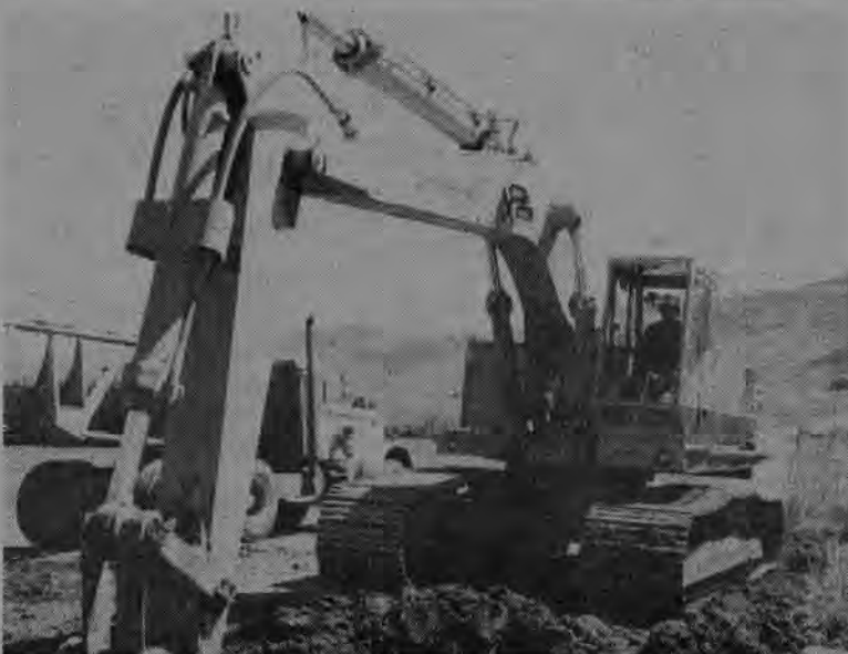
Pictured on the top photo on a backhoe is recently graduated apprentice Jack Isenberg, working for Helms Construction Co. Also operating a backhoe for Helms Construction on an underground project (bottom photo) is recently graduated apprentice Joe Woosley.
