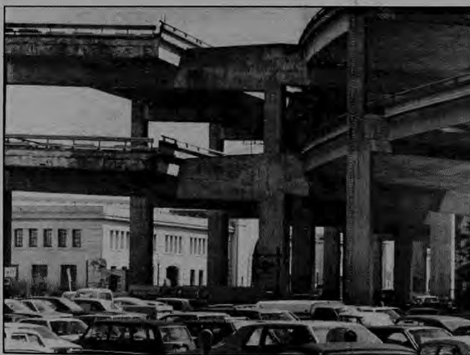
Embarcadero North Originally intended to skirt the north end of San Francisco and connect up to the Golden Gate Bridge, this freeway has remained unfinished for over a decade, and San Francisco officials vow it will never be completed. A move is now underway to tear down the entire stretch of Embarcadero Freeway and turn it into a street level, four-lane roadway.
