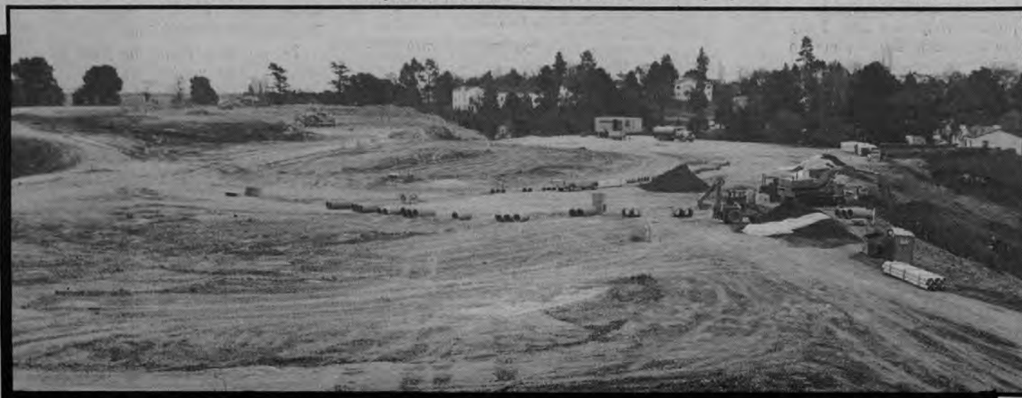
Kiewit-Pacific continues site work on housing project at Hamilton AFB.
