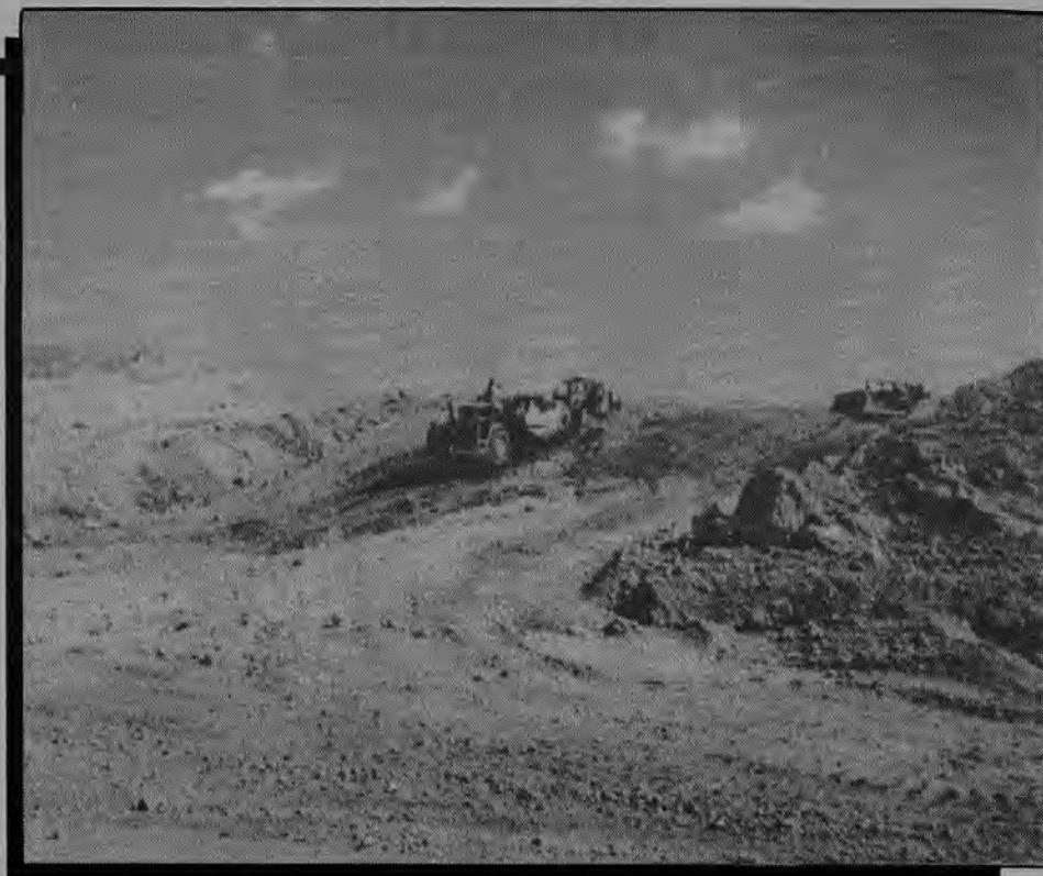
Local 3 member John Oliveira uses Cat dozer to push scraper operator Jesse Via on Korl Construction's West Beach job. Operating the other Cat is William Couch.
