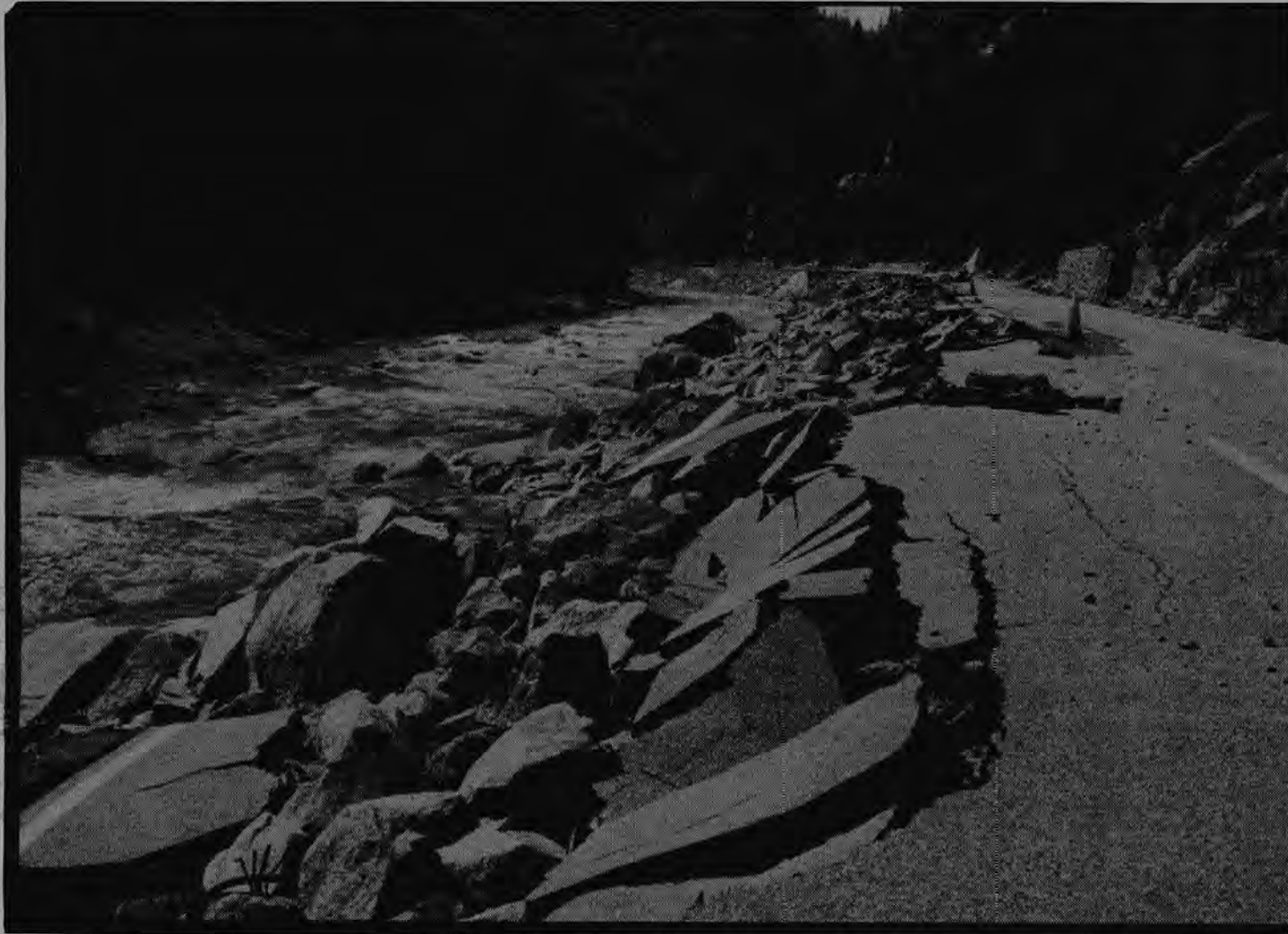
Over 20 miles of Highway 70 along the Feather River Canyon was ripped apart by flood waters.
