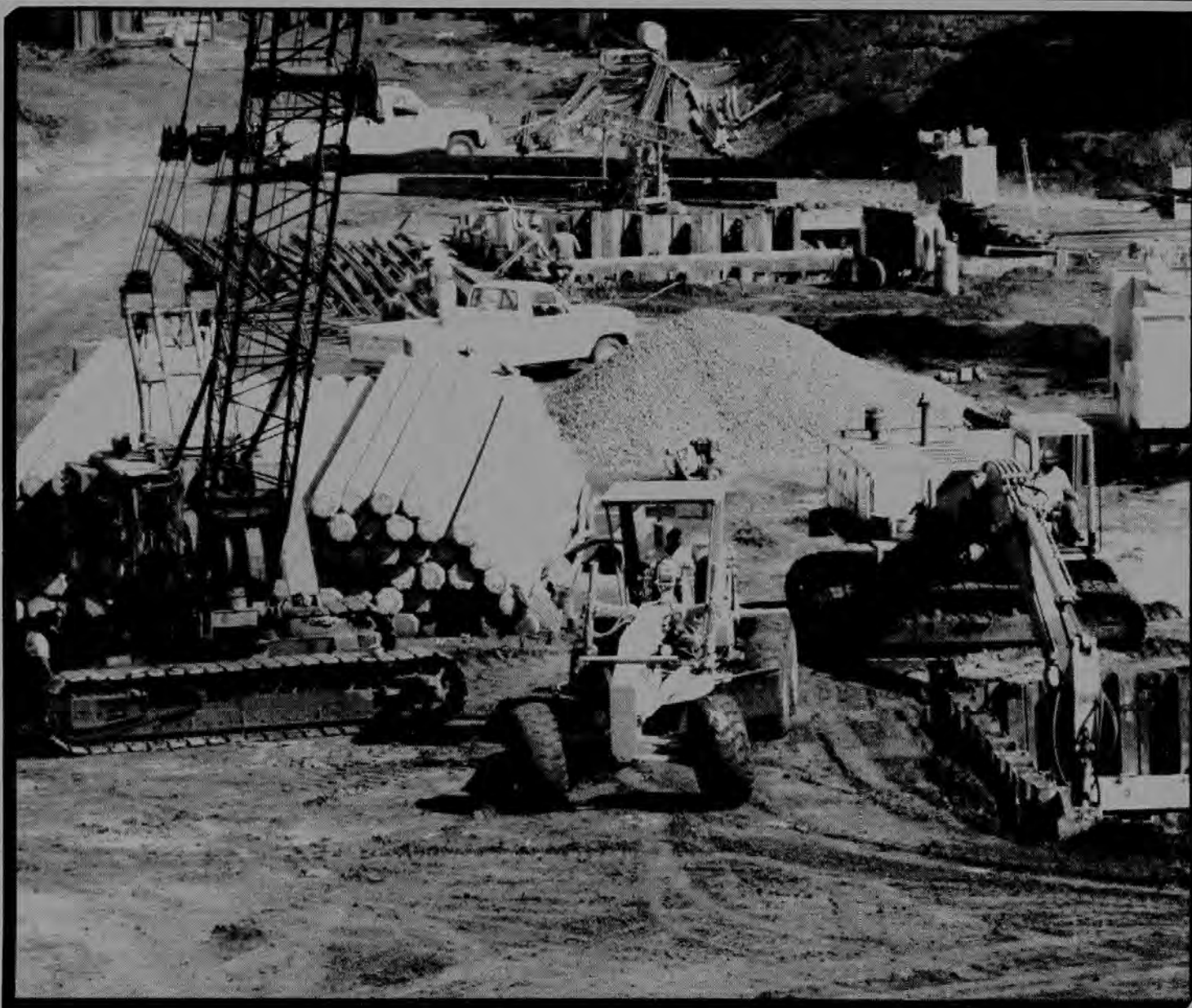
Pictured above are blade operator Sam Pa and backhoe operator Dennis Price working on the Hanamaula Bridge project.
