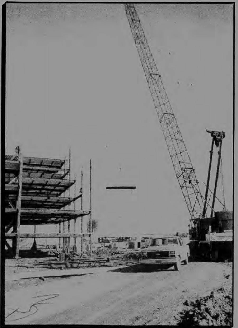
The main attraction of the 100-acre Metro Center of Foster City is this 22-story office complex being constructed by Rudolph and Sletten. Even though all the iron is not yet in place, the building is already 50 percent rented out.
