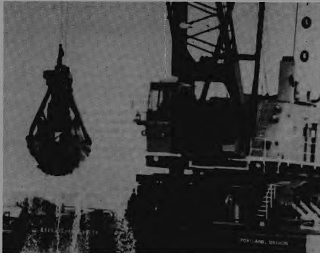
Pictured is the 'Big Dipper' owned by Riedel International of Portland, Ore. which worked two 10-hour shifts, six days a week for four months deepening the harbor at Crescent City. During this time, approximately 80,000 cubic yards of mud and rock was removed.
