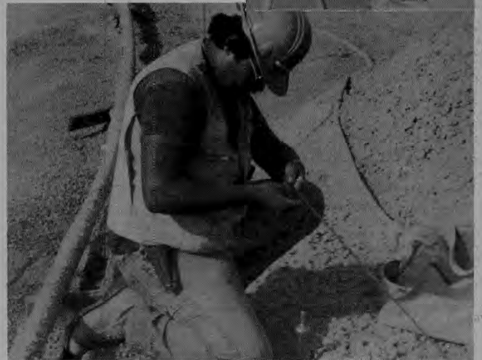
Pictured top right is Bill Webb, working on the PT&T job in San Ramon for Swinerton & Walberg. Bill has been a Local 3 member since 1955. Photo above shows third step apprentice Fabian Herrera working on Bill Webb's crew.
