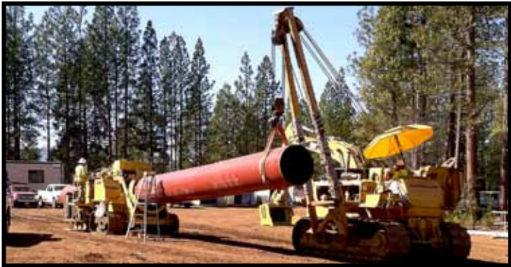
PAGE 23 In District 70, Pipeliner Zac Afong operates a pipe bender with the help of Pipeliner Sixto Morales operating a pipe layer. To learn more about summer work being done in the Redding District, including several bridge replacement jobs, read on.
