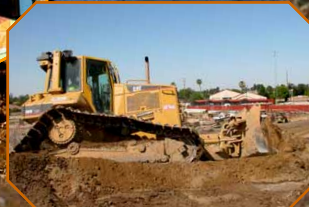
D6 Dozer Operator Mike Frithsmith dresses up the slopes.
