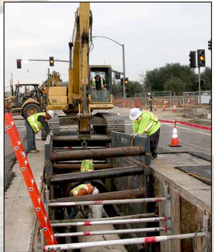
Excavator Operator Randy Cox puts a 60-inch, split-steel casing over a 36-inch water main on the Cosumnes River Boulevard extension job with Teichert.
