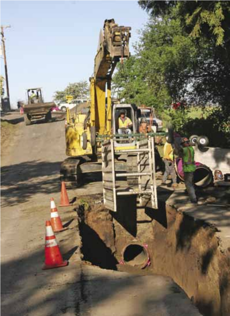
Excavator Operator Shon Cox places a cage in the ground so crewmembers can work on the shoring.
