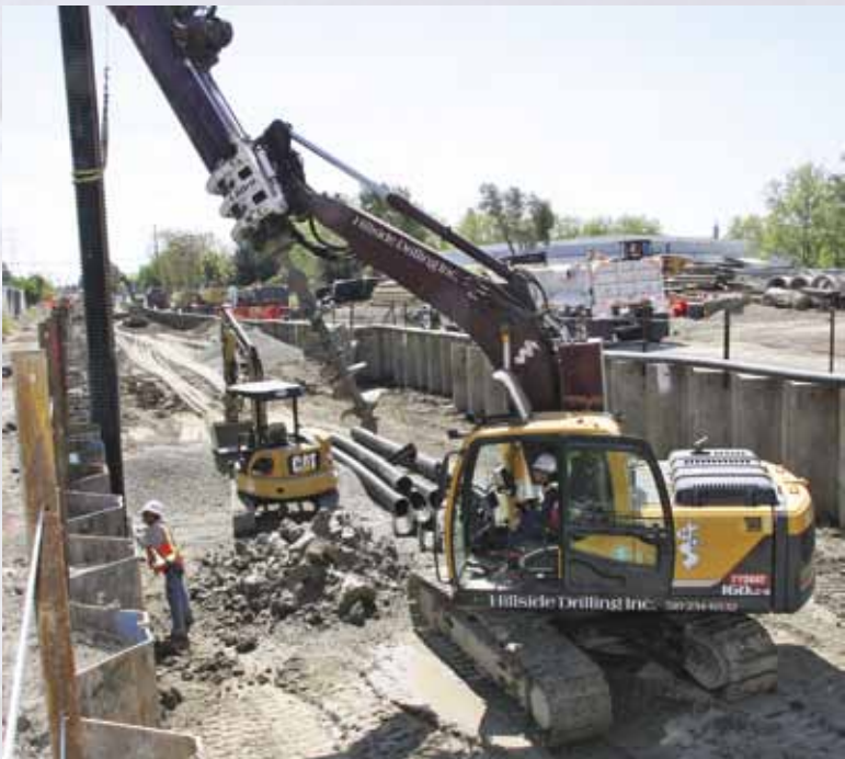
Operator Todd Carr digs wells for the Capitol jobsite using a lodrill.
