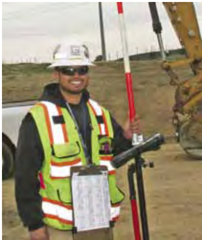
Francisco Garcia performs an as-built survey for Guida Surveying on the PG&E pipeline replacement job in District 80.
