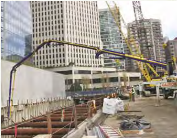
California Concrete Pump Operator Jose Moran pours out the bottom slab for the Transbay Transit Center project.
