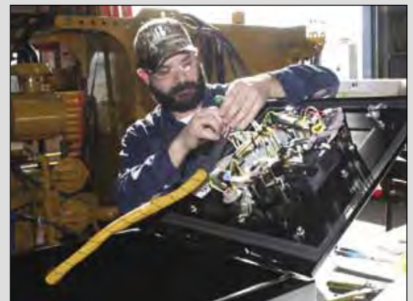
Field Service Technician Andy Bortolussi works on a control panel.
