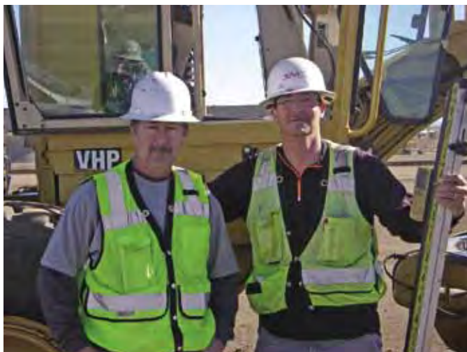
From Left: Blade Operator Michael Broersma and Gradesetter Steven Bouldin work at the Lemmon Valley warehouses for Sierra Nevada Construction.
