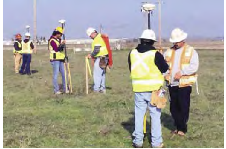
GPS students convert and stake the tree-mitigation plan for the new property.
