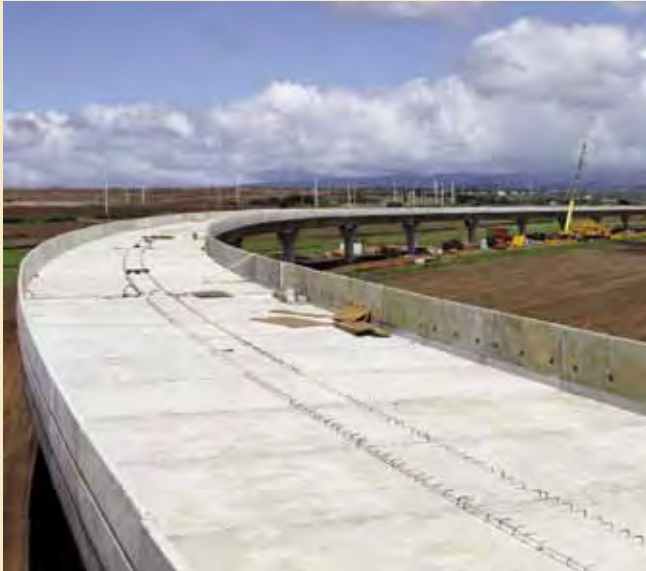
With each passing week, the rail guideway extends further east and west. Crews have erected more than 425 precast concrete guideway segments.
