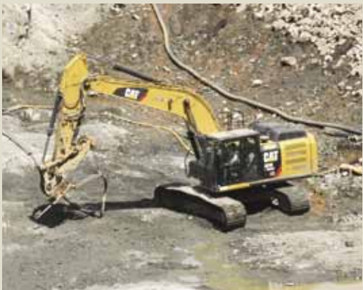
Excavator Operator Steve Fuller uses a high-power compressor to clean the bedrock while working on the diversion dike.
