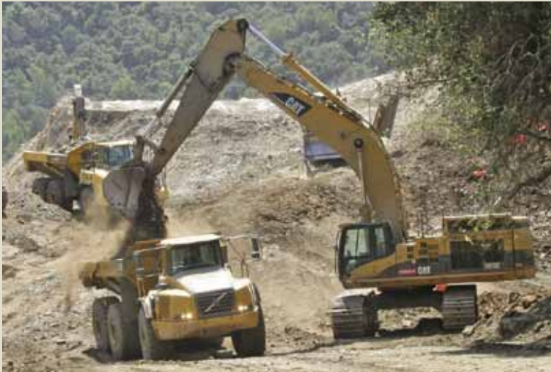
From left: Excavator operators Rick Gloege and Chris Baldwin load haul trucks with sediment to re-route the cut and alignment of the new river.
