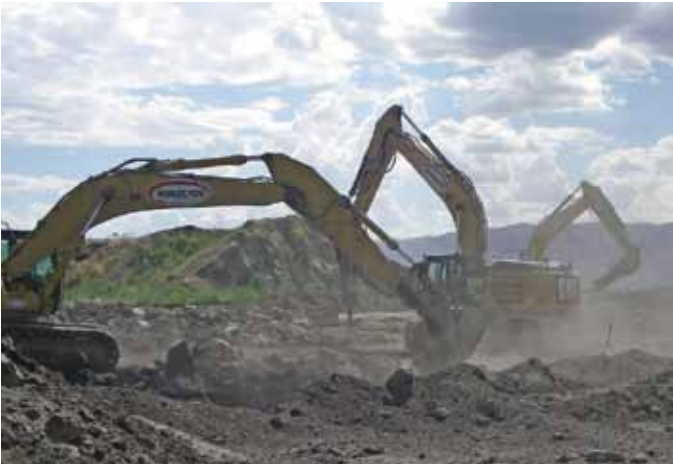
Members Jared Baxter, Jack Johnson and Bret McKendrick break and remove the underground concrete structures and foundations left from the Geneva Steel Mill for the Vineyard Connector project.
