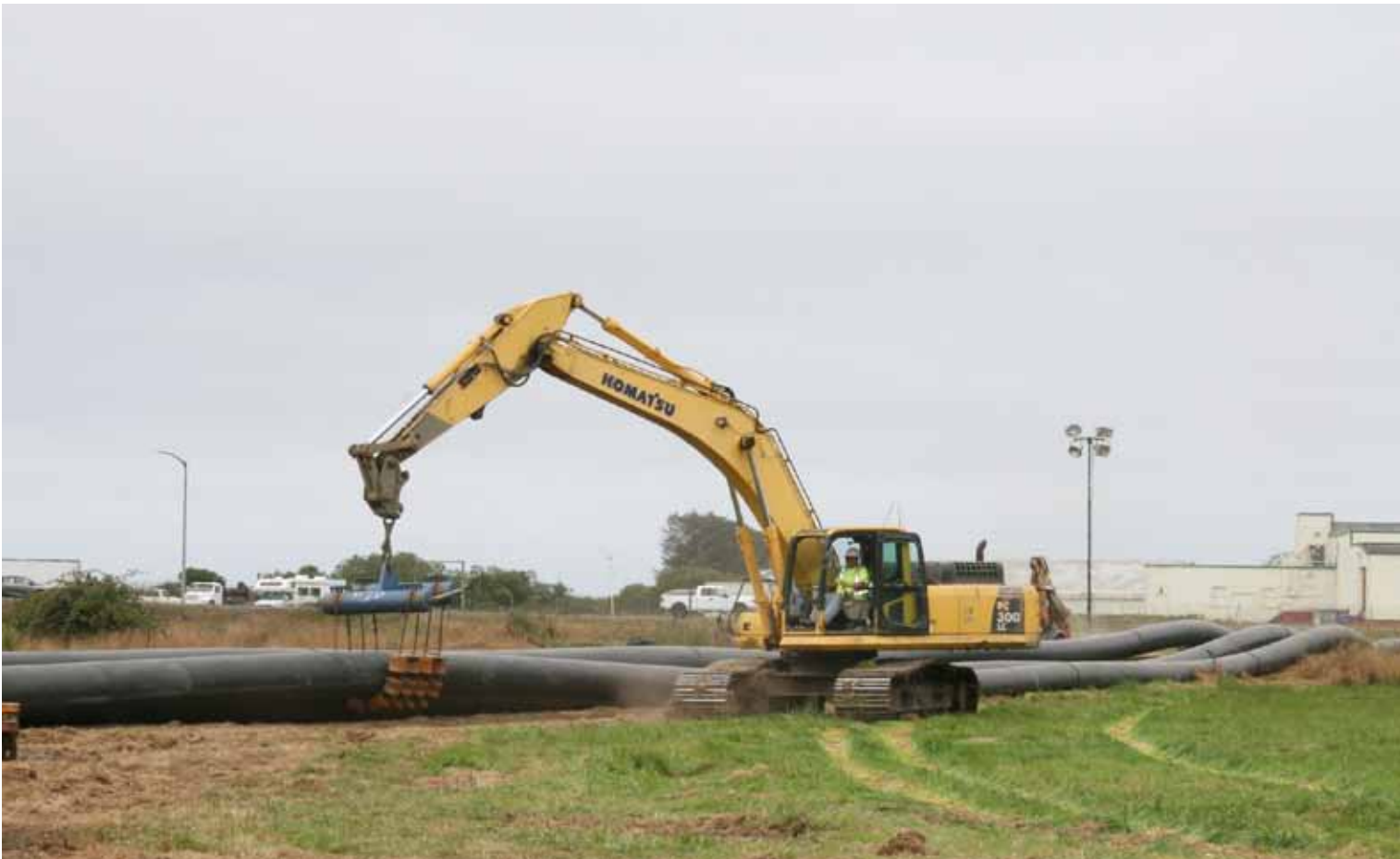
Excavator Operator Steve Warnow uses a saddle to stage the pipe so it can be pulled almost 4,500 feet to the other side of the job.
