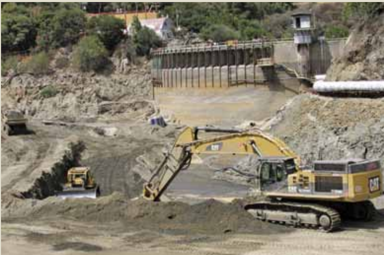
Dozer Operator Tommy Carrillo pushes the sediment on the river bottom toward Excavator Operator Travis Clements.
