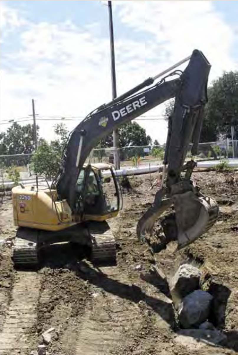
Excavator Operator Egidio Bettinelli artistically places giant rocks along the creek-bed to create pools for fish.
