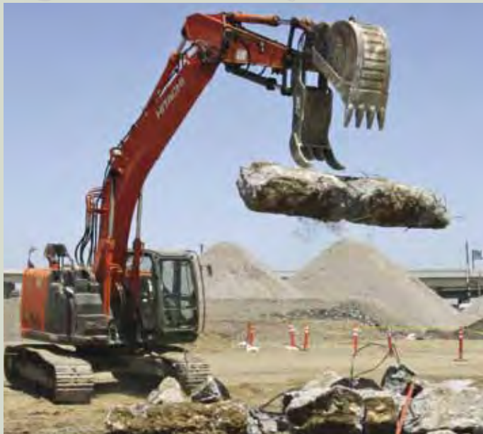
Excavator Operator Corey Bruce demolishes old foundations.
