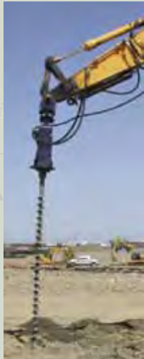
Third-step Apprentice Lillian Ferrer drills pre-holes at the old Oakland Army Base.
