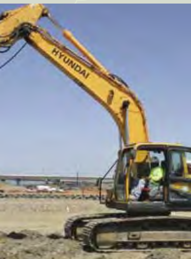
Richard Thornton drills pre-holes for the wick drains to be installed.
