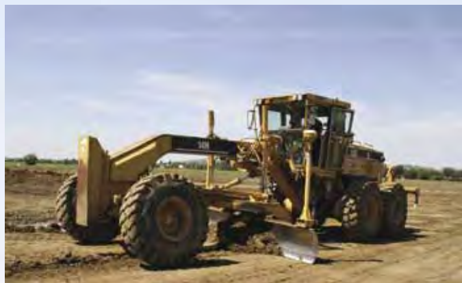
Blade Operator Robert Rust cuts pads on a 623-lot subdivision off Leisure Town Road in Vacaville.
