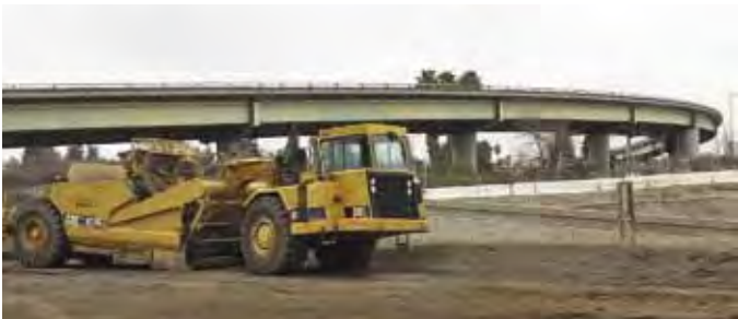
ABOVE: This photograph, taken by Retiree Gary Campagna in 1971, shows a TS14 Euclid scraper working on I-880 near Hwy. 17 in San Jose. BELOW: A scraper operator works in the same area along I-880 in San Jose in February.
