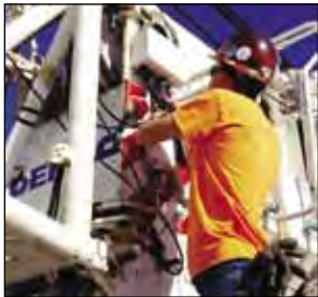
Apprentice Richard Kapushchinsky connects electrical wires for the luffing jib.
