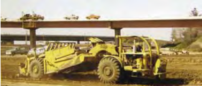
ABOVE: This photograph, taken by Retiree Gary Campagna in 1971, shows a TS14 Euclid scraper working on I-880 near Hwy. 17 in San Jose. BELOW: A scraper operator works in the same area along I-880 in San Jose in February.
