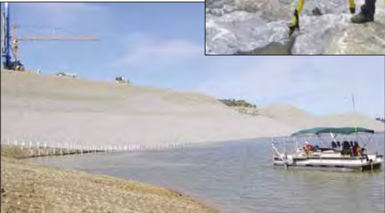
Working for R.E.Y. Engineers on the Folsom Dam auxiliary-spillway project, Matt Krueger, right, performs a terrestrial-scan survey of the step-chute, while a crew performs a bathymetric survey of the approach channel, below.
