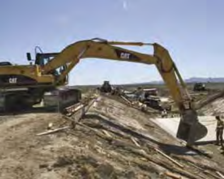
Excavator Operator Chris Coughlin and Gradesetter Trevor Meyers prepare to install 18-inch Reinforced Concrete Pipe (RCP) at the south end of the project.
