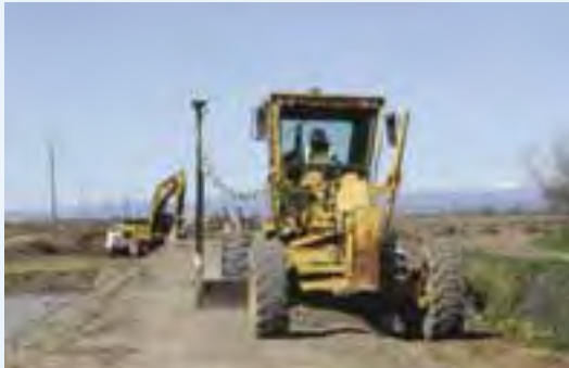
Blade Operator Rich Janc works along a portion of the canal that was widened by about 10 feet.
