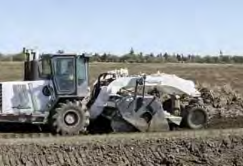
a stabilizer to mix the lime into material.
