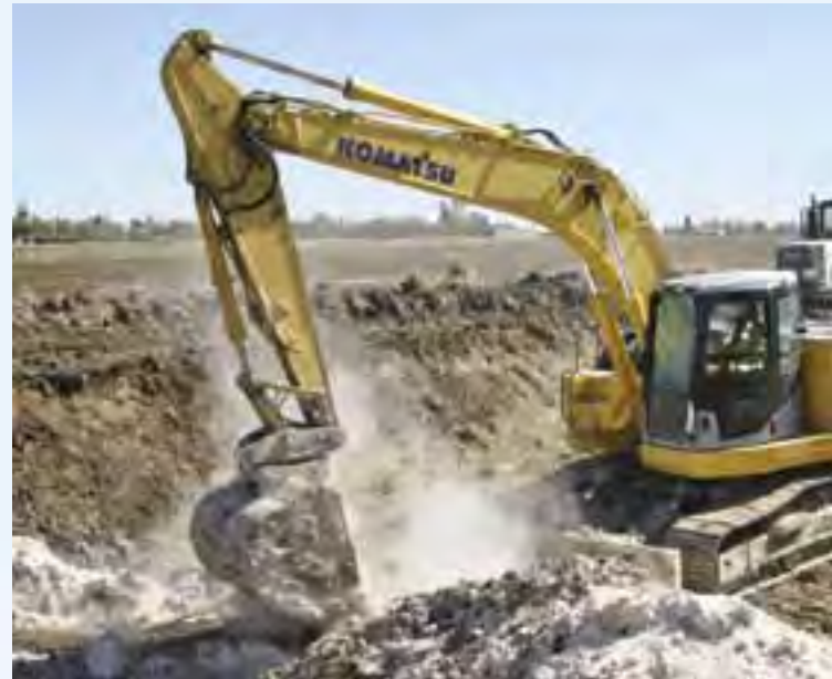
Excavator Operator Billy Mason uses his bucket to mix lime into the mud.
