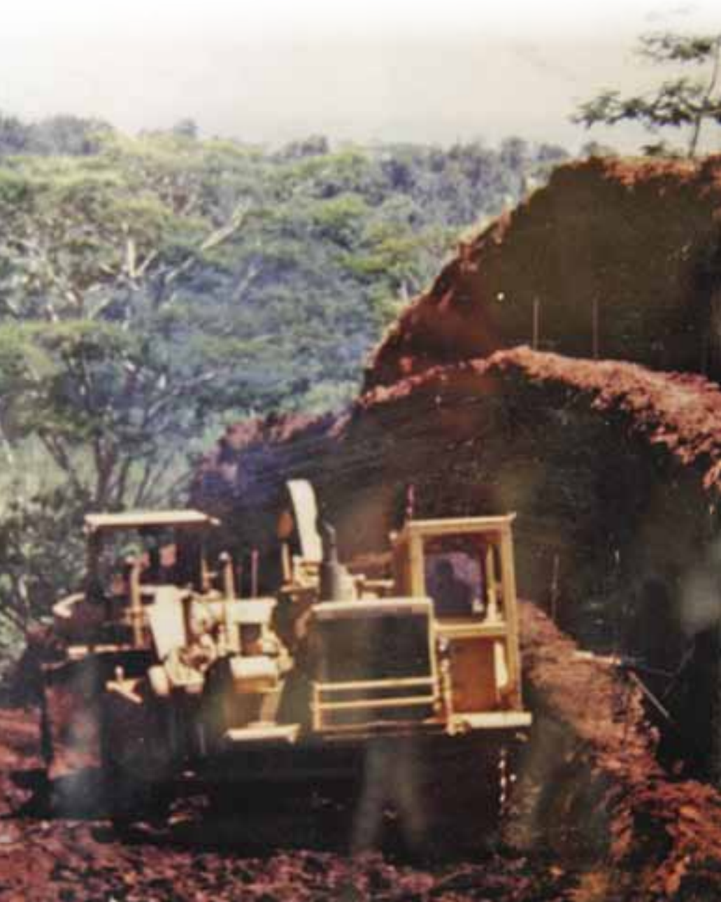
Retiree Joseph Sabala, above, works on the Kipapa Gulch, right, cutting a 1-½ to 1 percent slope to allow the trucks to go down and turn around.
