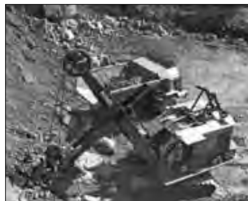
In 1965, member John Craft operates a Marion shovel to load an R30 Euclid truck at the Jackson Valley Reservoir project in Amador County.
