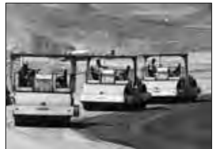
Compactor operators level the dirt on the giant Warm Springs Dam project in 1980.
