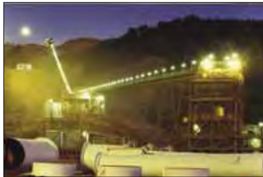
This 3,200-foot conveyor-belt system ran day and night on the Warm Springs Dam project and could handle 8 tons of material per minute.
