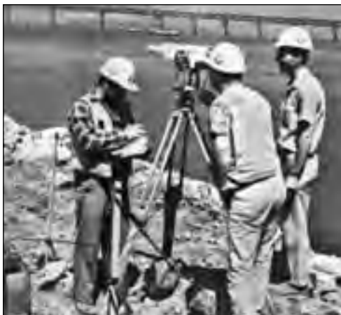
In 1967, Party Chief Dimitri Keriotis and surveyors Jerry Clow and Eugene Schaufler set up laser beams for aligning the huge BART Transbay Trench.
