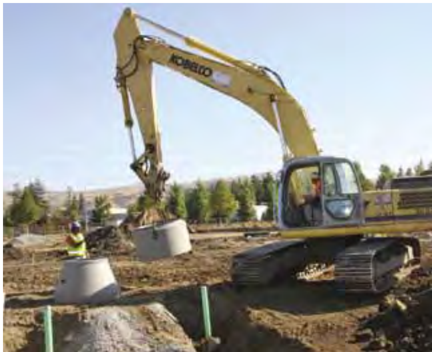
Mountain Cascade Excavator Operator Kristian Anderson sets pre-cast for sewer manholes.
