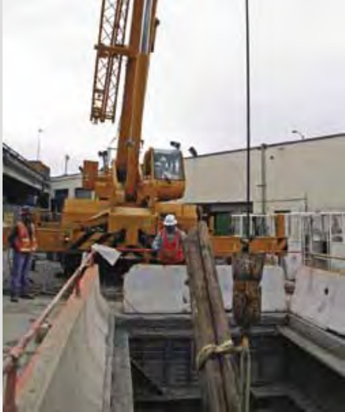
Crane Operator Paul Breaux lowers supplies to the mechanics inside the tunnel through opened sections of roadway.
