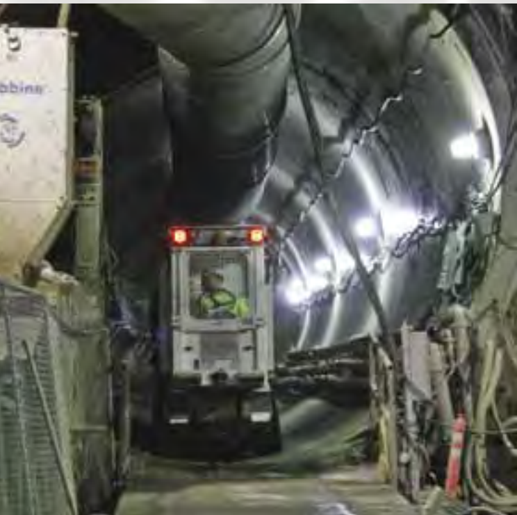
TBM Mechanic Kory Sepulveda catches a ride on the Tunnel Service Platform (TSP) that takes workers in and out of the southbound tunnel.
