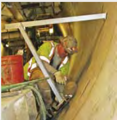
Mechanic Steve Wagerman installs brackets for the conveyor belt that will eventually take rock and muck all the way from Chinatown to the jobsite off Harrison Street.
