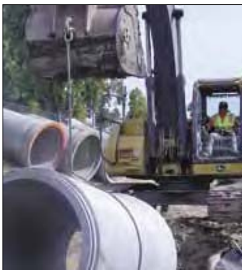
Excavator Operator Miguel Figueroa works with a 42-inch drain pipe for Team Ghilotti at Lake Dalwigk in Vallejo.
