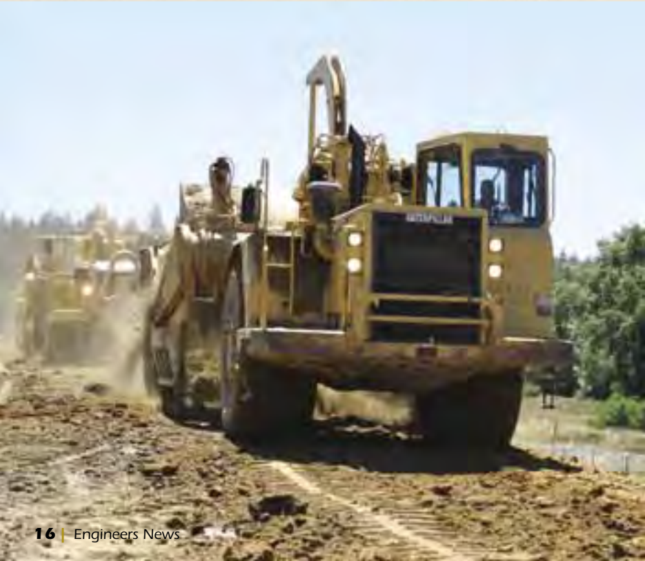
Scraper operators Robert Silva and Miles Robinson move some of the 1 million yards of dirt on the grading portion of the project.
