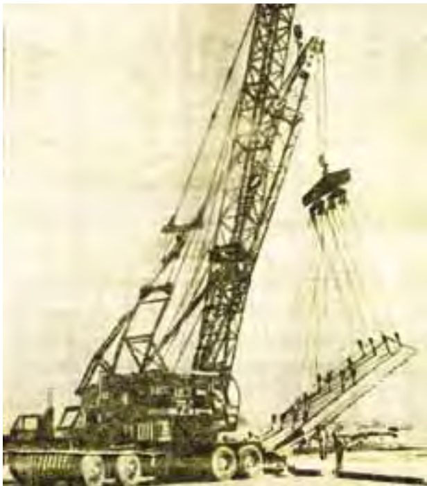
In November 1961, Local 3 operators use two heavy-duty truck cranes to erect “some of the heaviest precast concrete-wall panels ever used,” at 45 tons each, on a jobsite in Davis, Calif.
