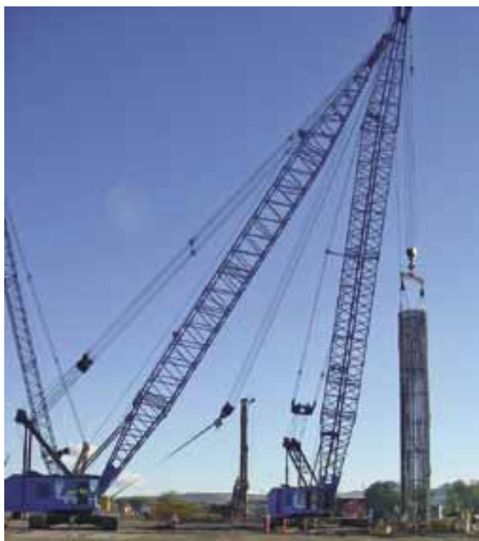
Operator Charles "Chuck" Neller Jr. , Oiler Ricardo "Rick" Fernandez and Apprentice Chelsie Greywolf set column cage on the first phase of the South East Connector project for Case Foundation.
