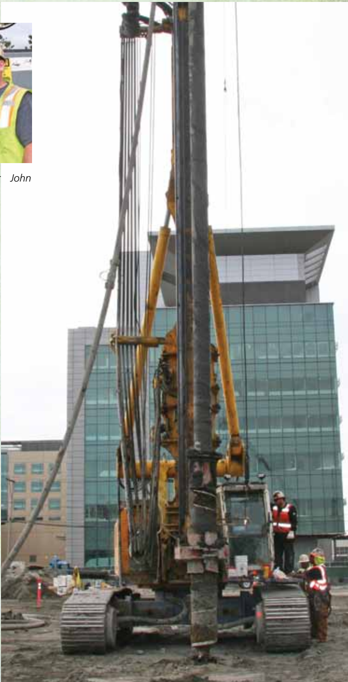
Berkel Drill Operator Donald Card drills piles for a UCSF Medical Center office building.
