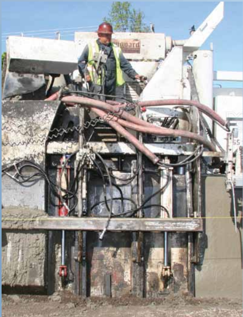
Miller Machine Operator Jose Aguilar creates the center divide on Hwy. 99 for Vanguard Construction.
