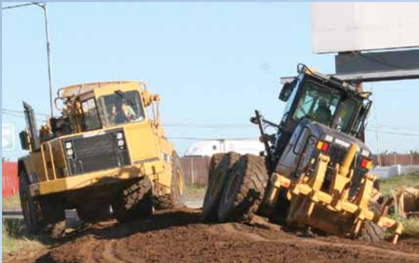
From left: Scraper Operator Jason Jackson helps Blade Operator Tony Arnaiz, also on cover, fill the chokers and compact the dirt.
