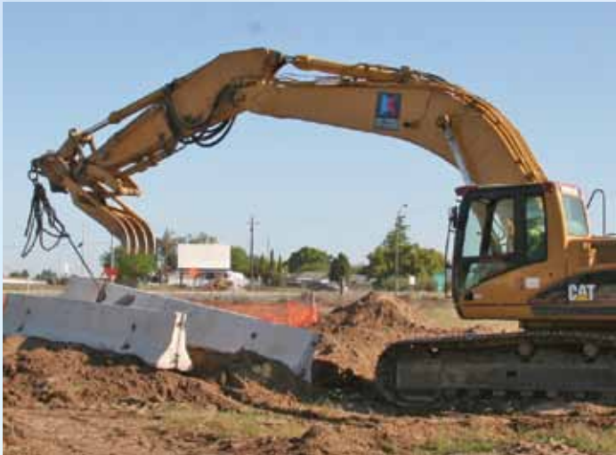
Excavator Operator Jose Garcia moves K-Rail into place along Hwy. 99.
