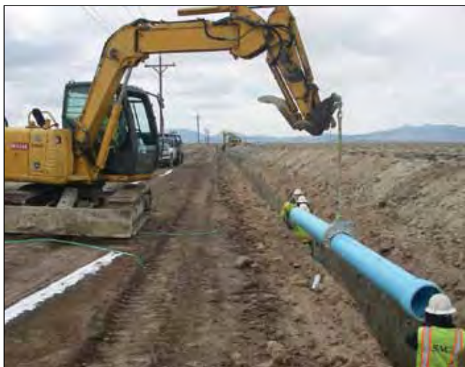
Excavator Operator Frank Higgins sets pipe for Sierra Nevada Construction on a waterline project in Austin.
