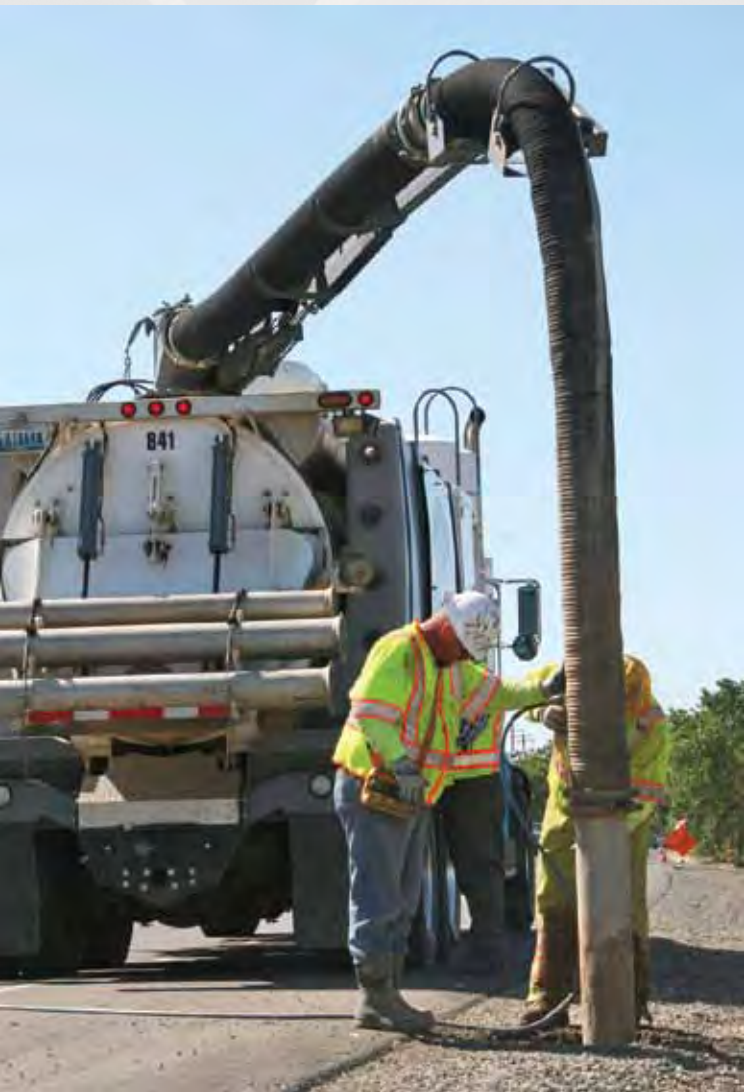
Hydro-vac Operator Jason Bell performs potholing for Badger Daylighting.
