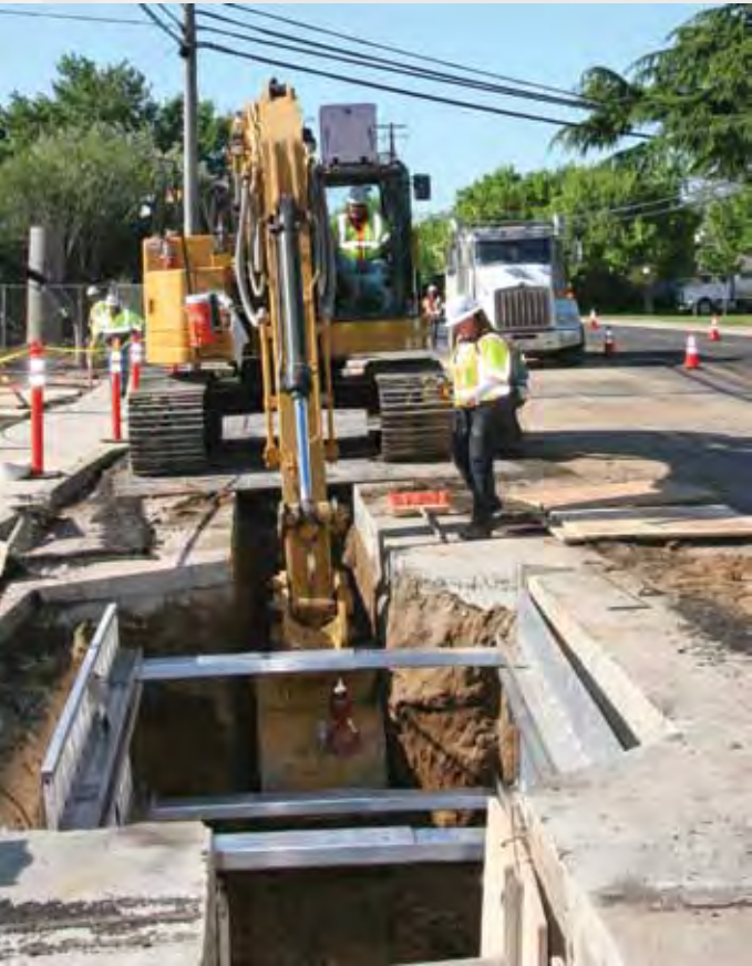
Excavator Operator Kevin Butler and Oiler Carla Estes put in a shoring box for a tie-in.
