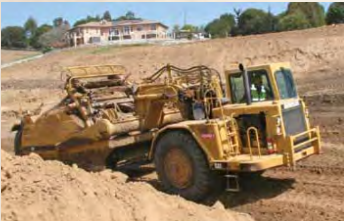
Paddlewheel Scraper Operator Shawn Ogan delivers some of the 250,000 yards of dirt moved for the Hwy. 101 San Juan Road interchange job.
