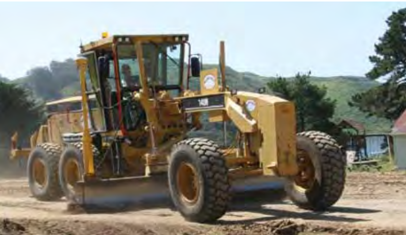
Blade Operator Sam Vassey utilizes GPS while working on a new parking lot for the Marine Mammal Center.
