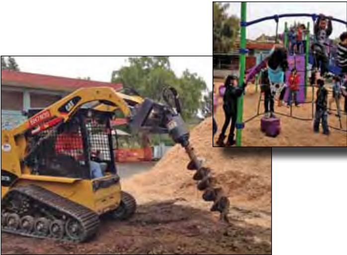
Skid-steer Operator Jason Kenyon uses an auger bit to drill holes for playground equipment in Hayward.
