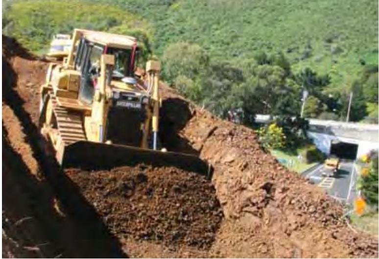
Dozer Operator Lee Montenegro creates a rock catchment for Maggiora & Ghilotti, Inc.
