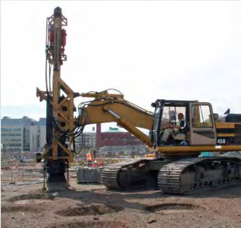
RIC Machine Operator Greg Winters improves the soil for roads on blocks 11 and 13.
