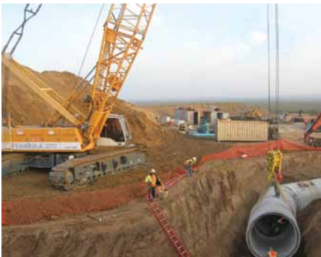
Crane Operator Paul Maddox and Oiler Jake Raine set 96-inch pipe for Mozingo Construction.
