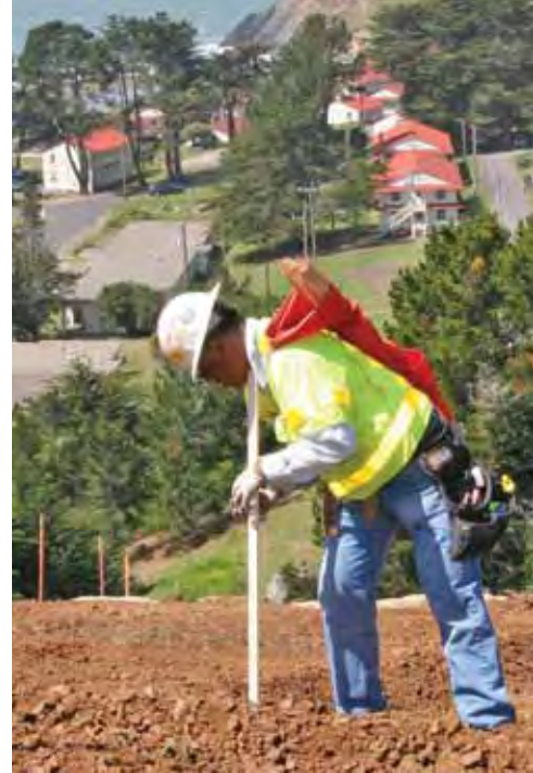
Gradesetter Tim King performs some slope-staking, as operators return the old Fort Cronkhite Parade Ground Quarry to its original state.
