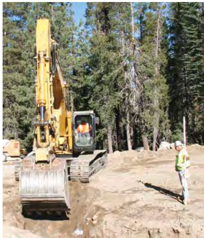
Excavator Operator Shawn Broyles and Gradesetter Steve Leal work on the footing for a tank pad.
