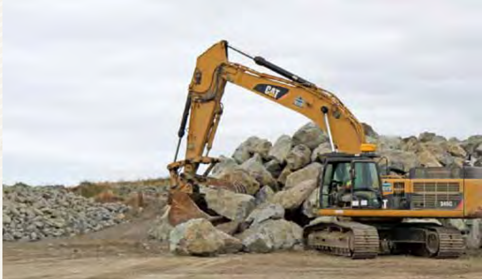
Six-year member Curtis Booth stages the rock that will be used on the slopes surrounding the inner-boat basin. There are three different classes of rock being used, including the backing rock (at left), quarter-ton rock (not shown) and 2-½-ton rock (at right), which will be used on top.
