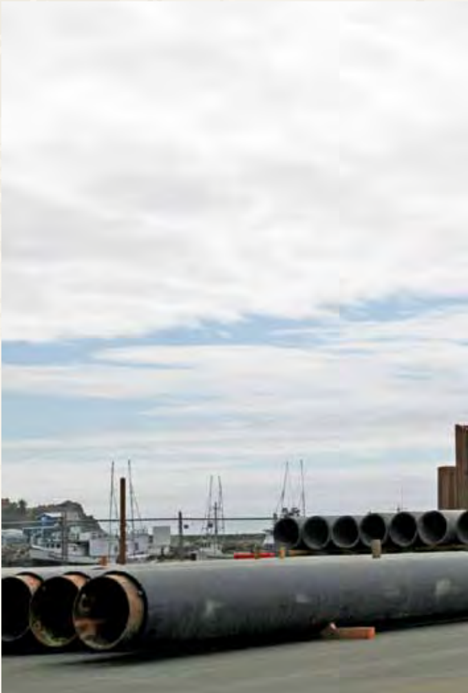
Dutra adds high-density polyethylene sleeves to the pilings that are staged at the harbor. The sleeves are part of the new design and will protect against corrosion.
