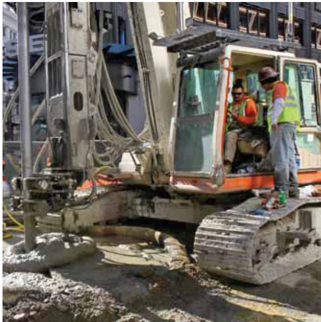
Rustom Ebalo and Ryan Federighi perform jet grouting for the Central Subway project.
