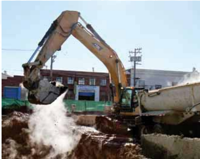
Excavator Operator Lisa Anderson fills eight to 10 trucks a day with jet-grout spoils for Barnard.
