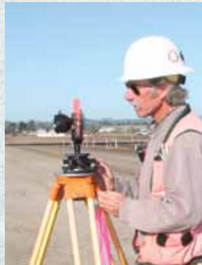
Chainman James Glendening works on gridlines for the parking-lot structure on the Graton Rancheria Casino Resort and Hotel project.
