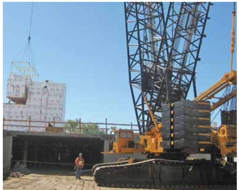
Bragg Crane Operator James Hudgins and Oiler Michael Lepiane use a Liebherr 1400 425-ton crawler to make a 68,000-pound lift.
