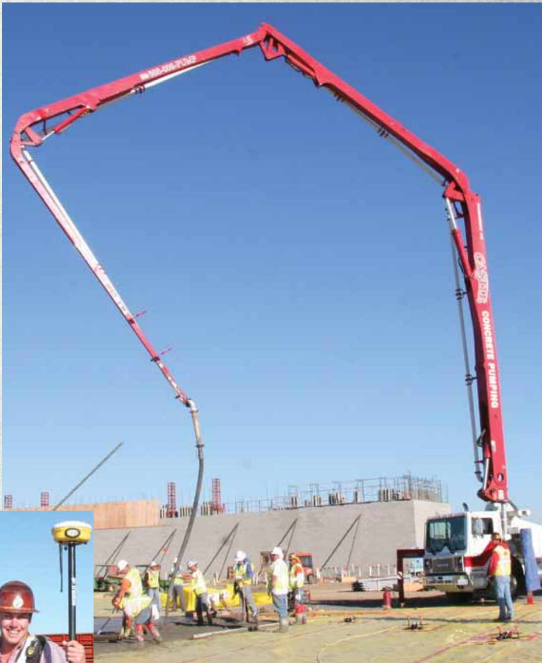
Concrete Pump Operator Emil Bacigalupi makes a pour for the slot-machine area.
