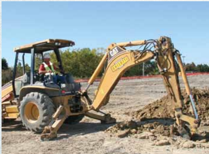
Backhoe Operator Jerry Reiter works on the subdrain for the spillway overflow on the Graton Rancheria Casino Resort and Hotel project.
