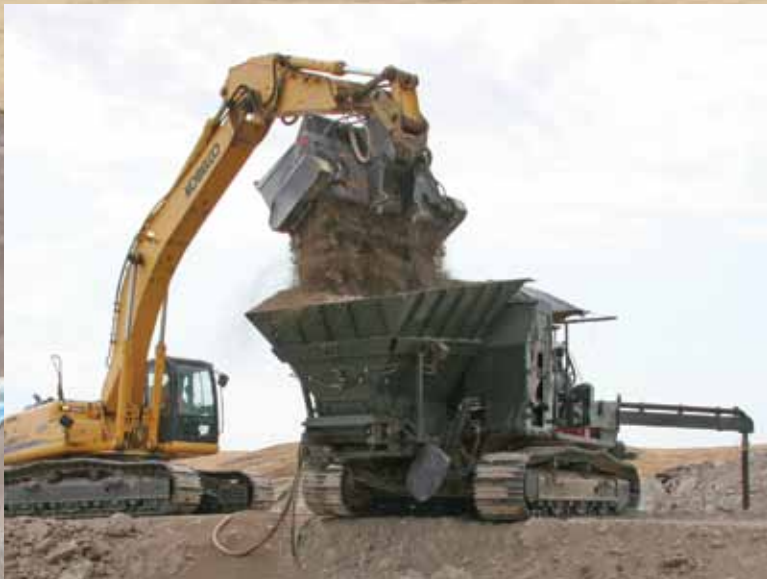
Blue Iron Excavator Operator Marcial Fernandez uses a screening bucket to drop material into the slurry machine.
