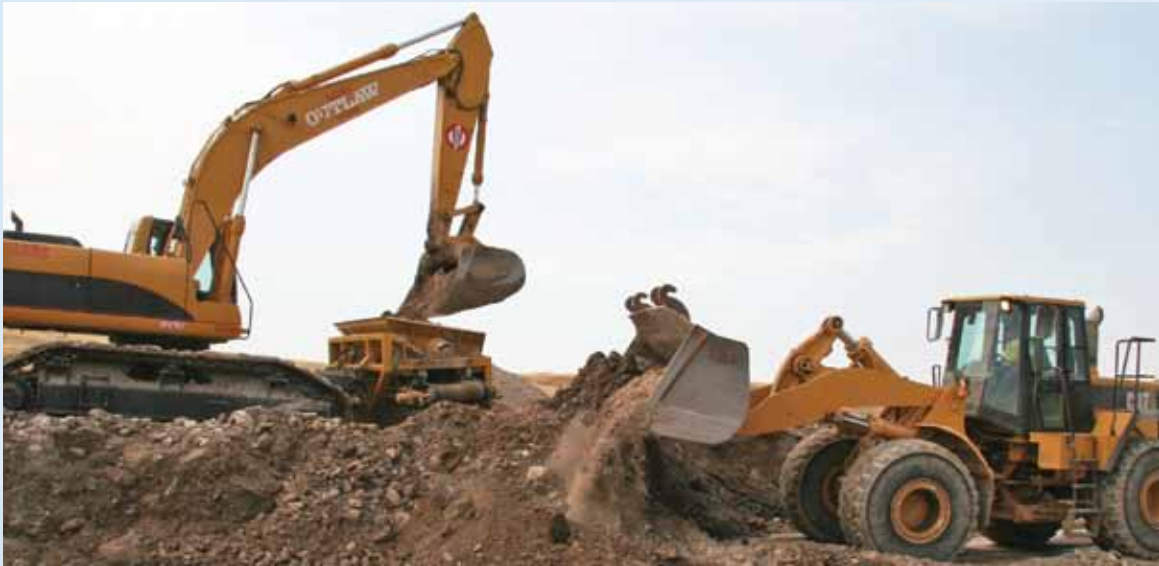
From left: Excavator Operator Mike Gross drops rock from Loader Operator Ron Muntz into a screener, or “grizzly,” to be used for backfill.
