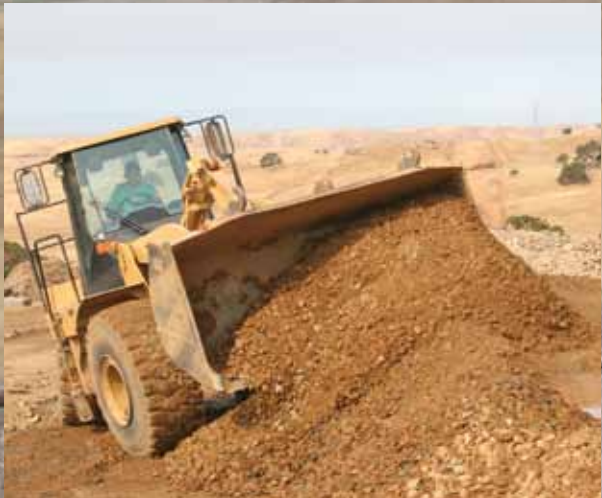
Loader Operator David Tonegato backfills the newly laid pipe.
