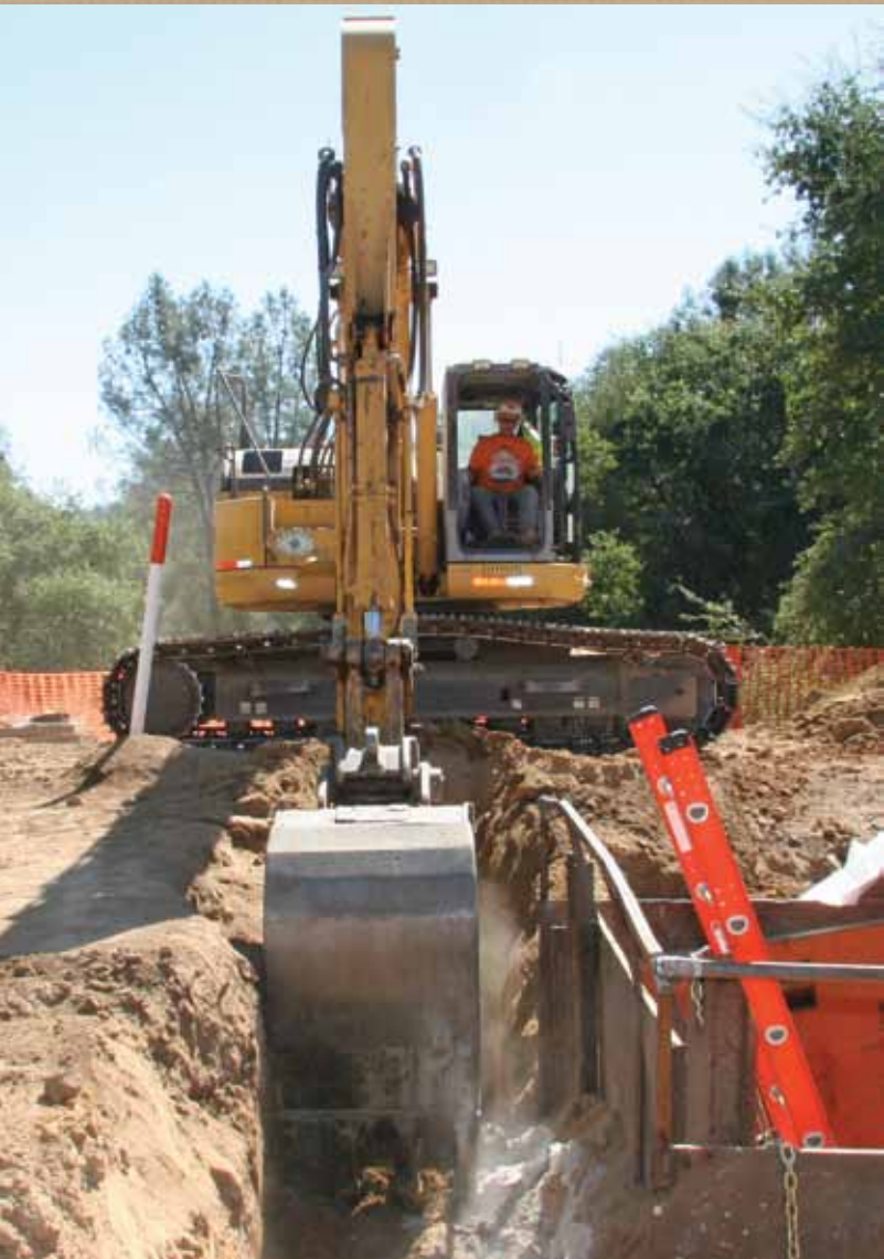
Excavator Operator Ron Lorance removes cement from a bore pit.
