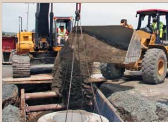
From left: Excavator Operator John Escobar removes a trench shield with help from Loader Operator Kawika TaVares.
