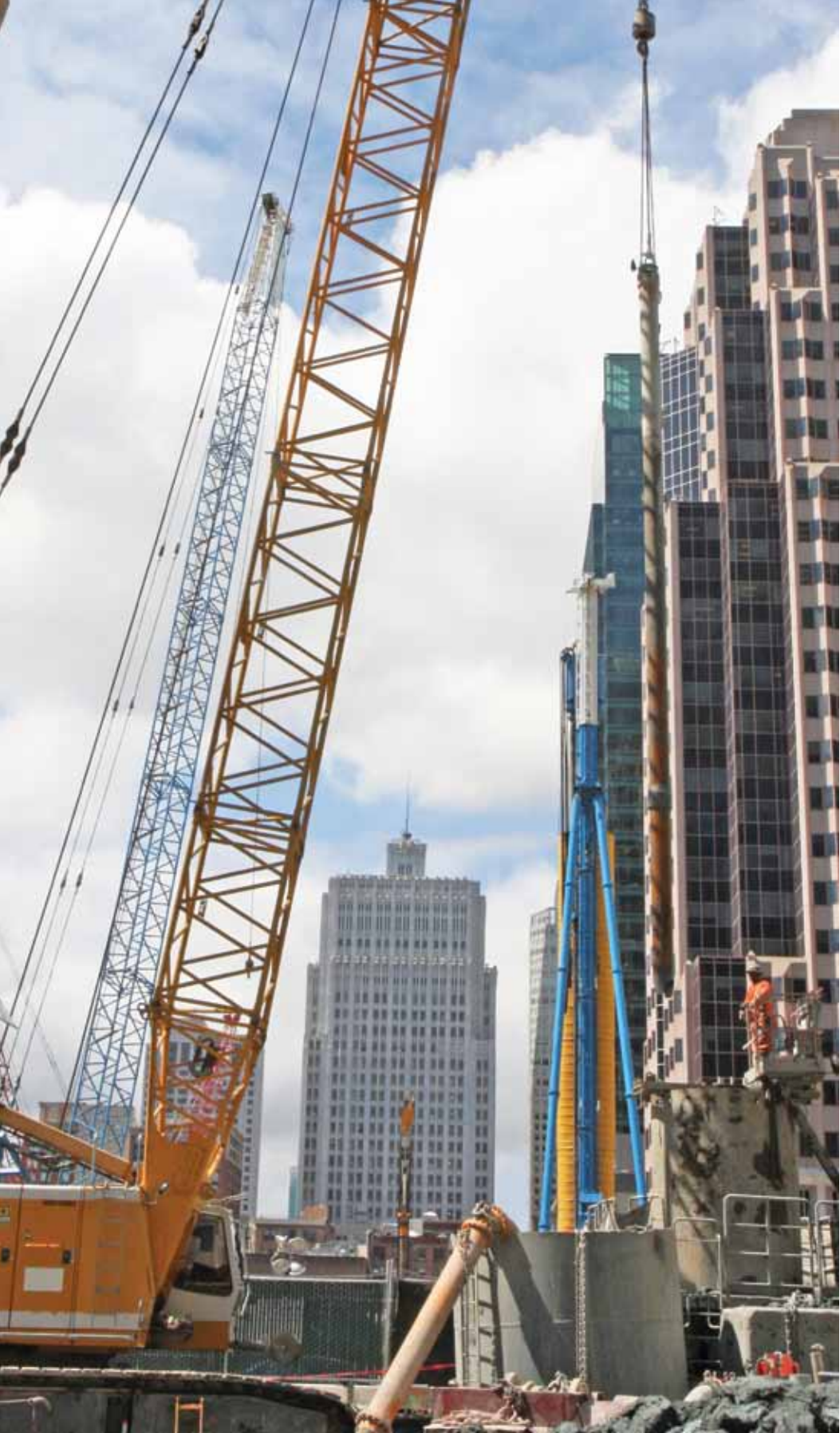
Crane Operator Mark Powell and Darren Crawford (on manlift) add a section of tremie pipe for the concrete pour.
